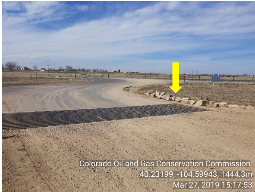
Photo 19 Inadequate tracking pad BMP
