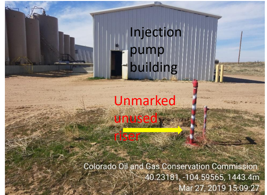
Photo 16 Unused unmarked riser
