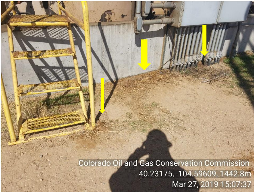
Photo 13 Stained soil around active injection battery
