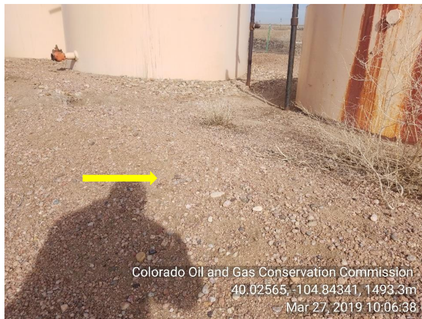
Photo 3 Inadequate berms
