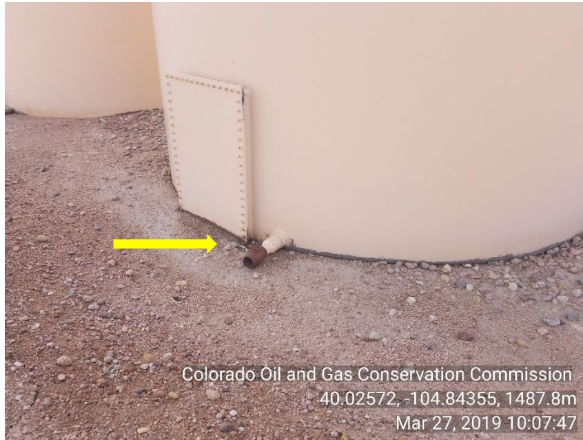
Photo 7 No bull plug load line crude oil tank
