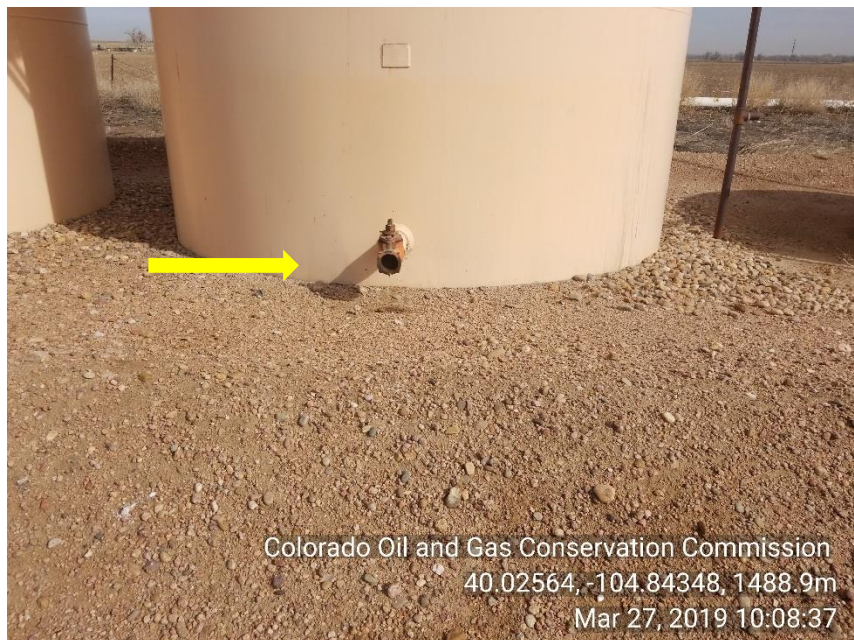
Photo 9 No bull plug load line crude oil tank
