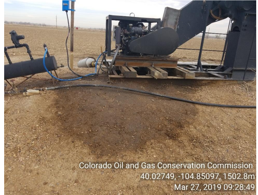
Photo 2 Stained soil around PU motor
