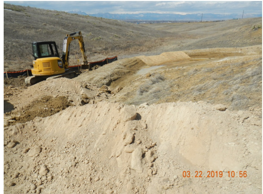
Photo 6. Photo taken from the western perimeter of the location, facing South. Appears the Operator has installed a sediment trap with a temporary stabilized outlet.
