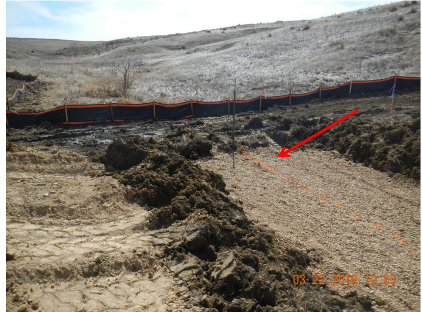
Photo 4. Photo taken from the southern perimeter of the location, facing Southeast. Appears the operator is installing a culvert through the USFWS National Wetlands Inventory mapped Riverine System (R4SBC).
