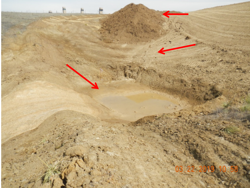
Photo 9. Photo taken from the western perimeter of the location, facing North. The middle ground of the Photo depicts erosion observed on location with apparent sediment accumulation within the sediment trap. The background of the Photo illustrates the topsoil stockpile has not been temporarily stabilized.
