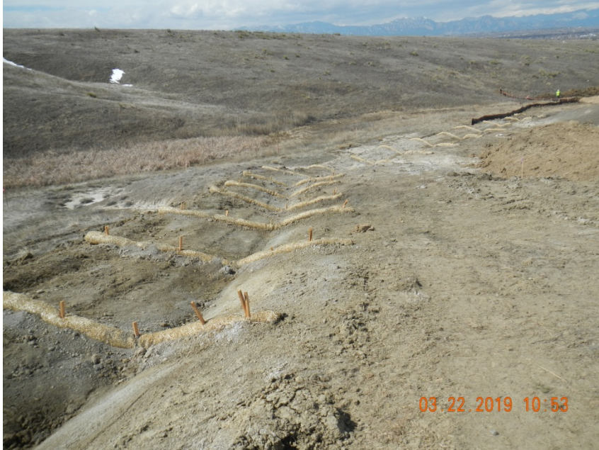
Photo 1. Photo taken from the southern perimeter of the location, facing West. Photo illustrates a ditch and berm BMP that is being installed around the perimeter of the location.
