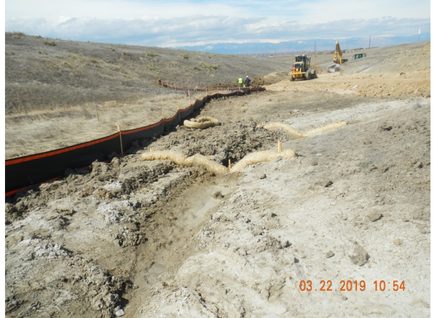
Photo 2. Photo taken from the southern perimeter of the location, facing West. See comments from Photo 1. An additional silt fence BMP is installed on the southern edge of the location.
