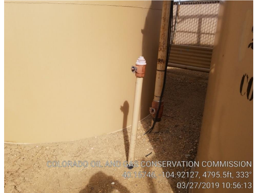
Pic 6 Unused unmarked riser
