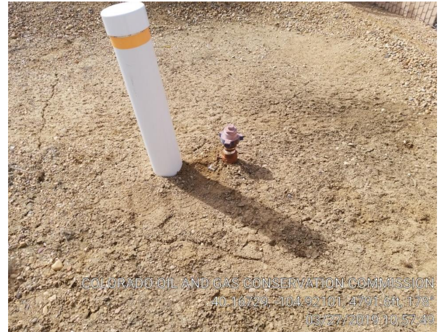
Pic 8 Unused unmarked riser
