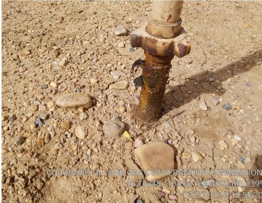
Pic 5 leaking riser in tank battery.
