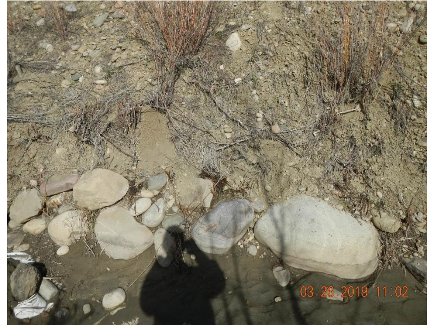
Residual impacts along High Flume siphon bypass.
