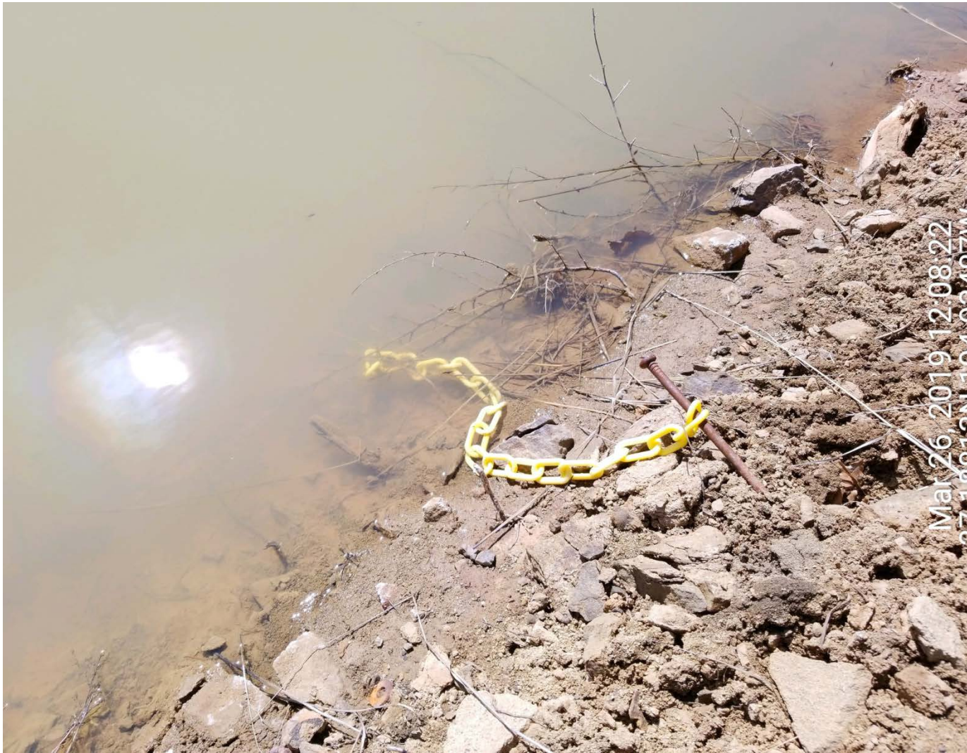
Freeboard marker is submerged.
