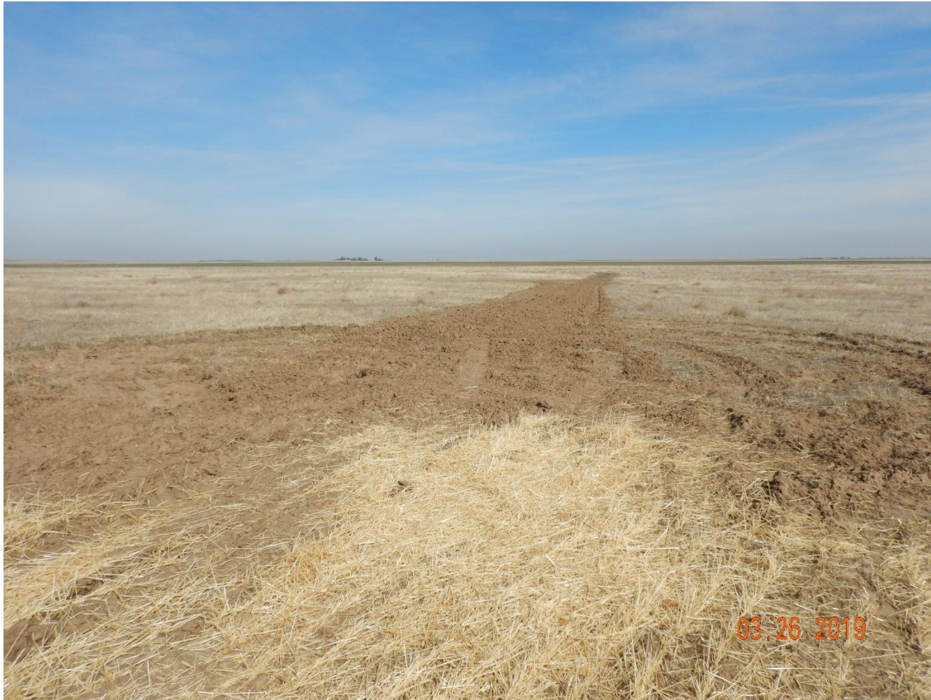
Photo 2: Photo taken from the section of access road within cropland, facing north. Photo shows additional reclamation activities have been conducted along access road. Photo also shows utility poles have been removed from location/access road.
