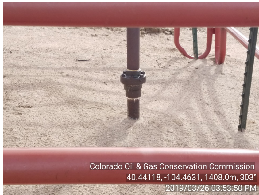
Photo #4 State 23-32 Wellsite Unused riser - Removed
