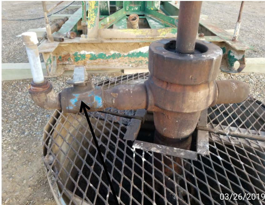
Photo 5. Casing valve leaking gas.
