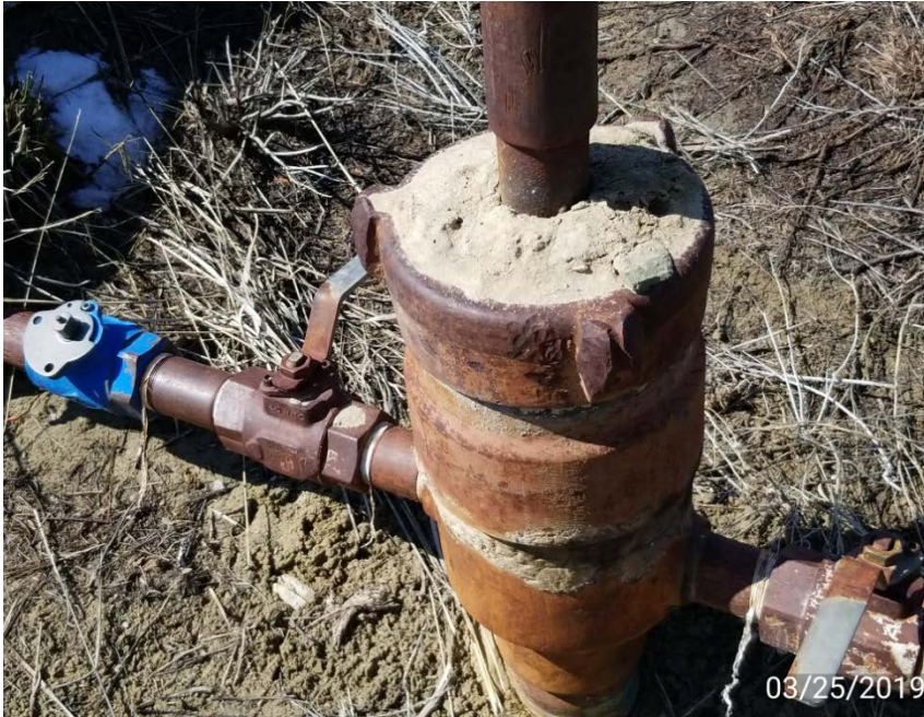
Photo 3. Well head leak.
