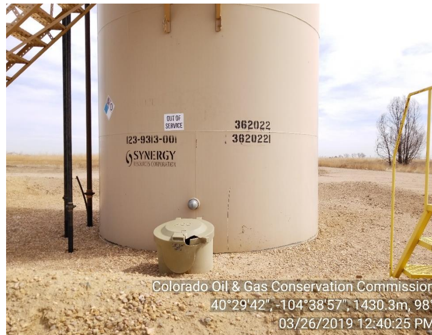
Photo 4: Inadequate labeling on tank.
