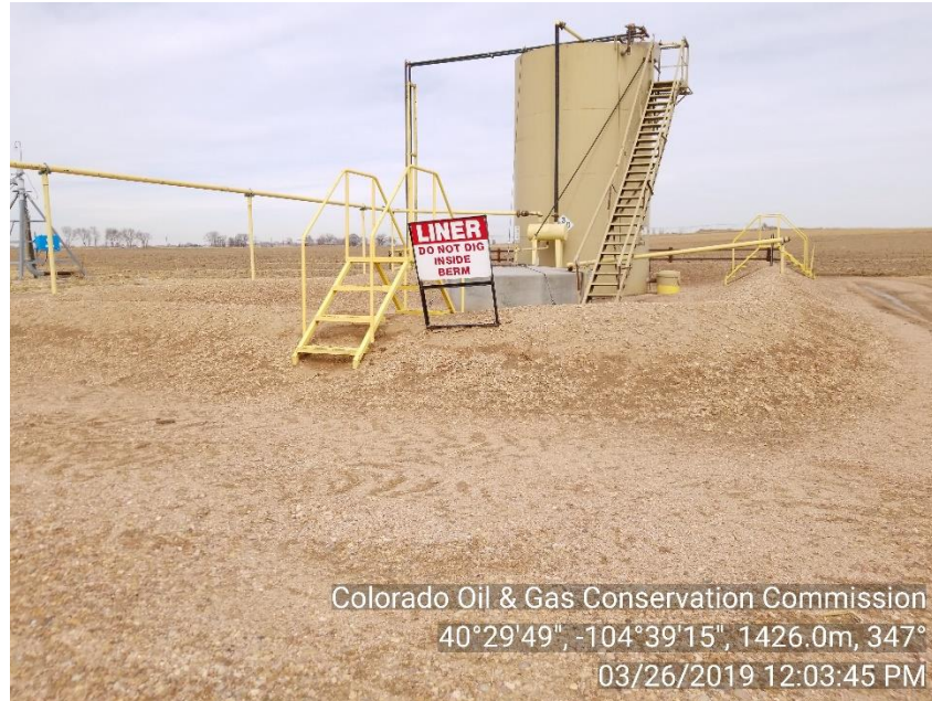
Photo 3: Incorrect berm around tank battery
