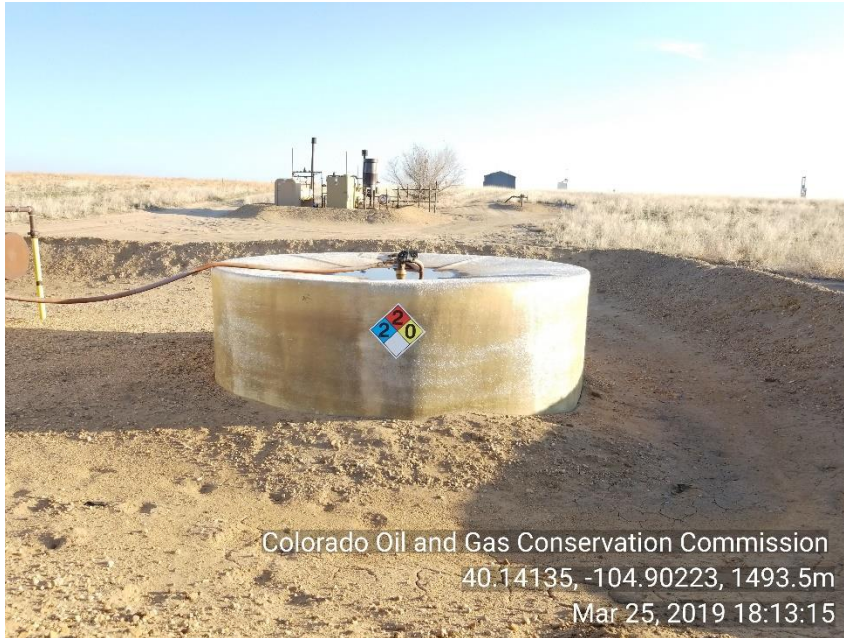
Photo 5 produced water tank no volume placard or identifying placard
