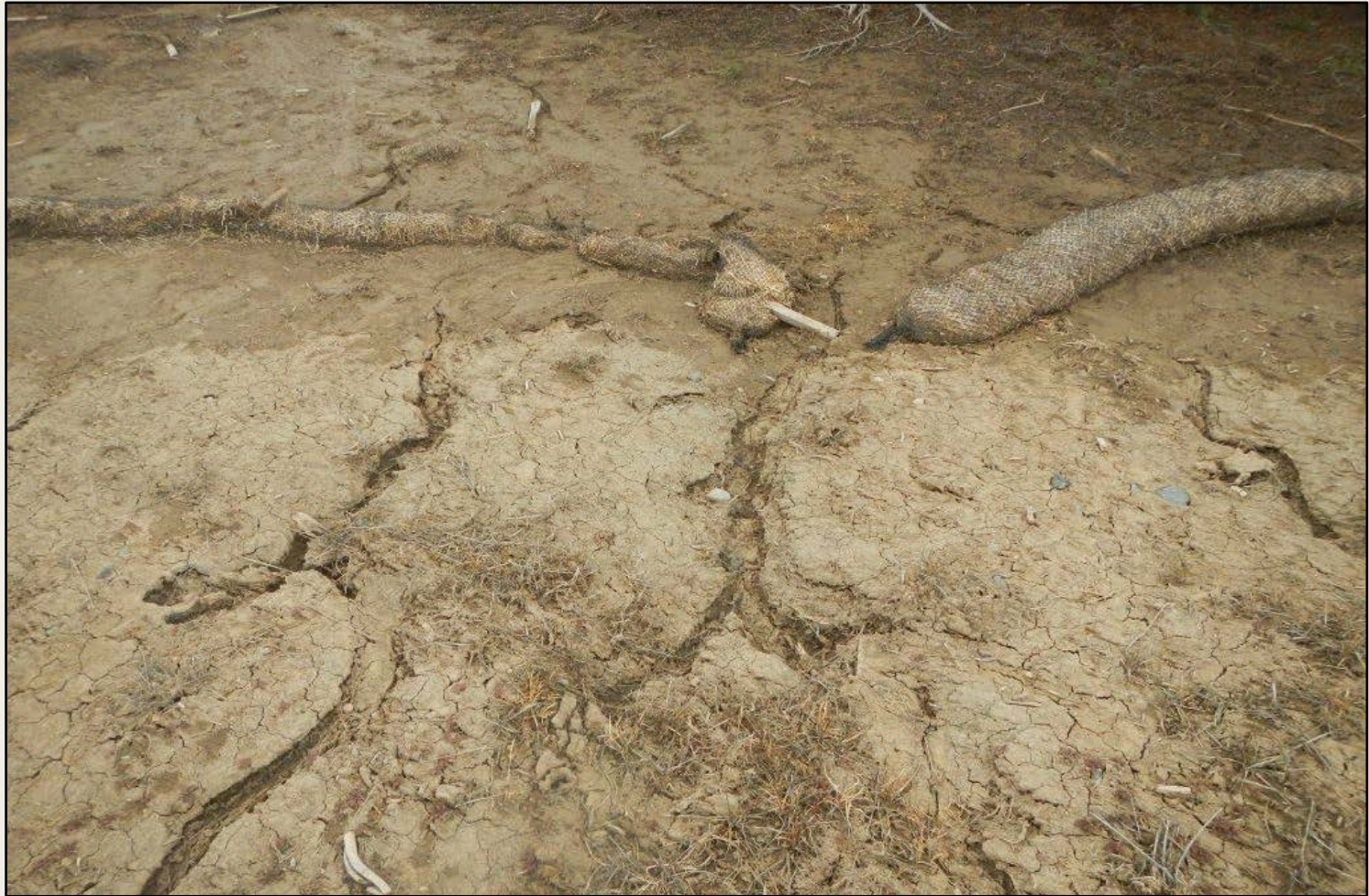
Photo 4. View of more erosional channels showing failed wattles and sediment deposition offsite, within the southern project area.
