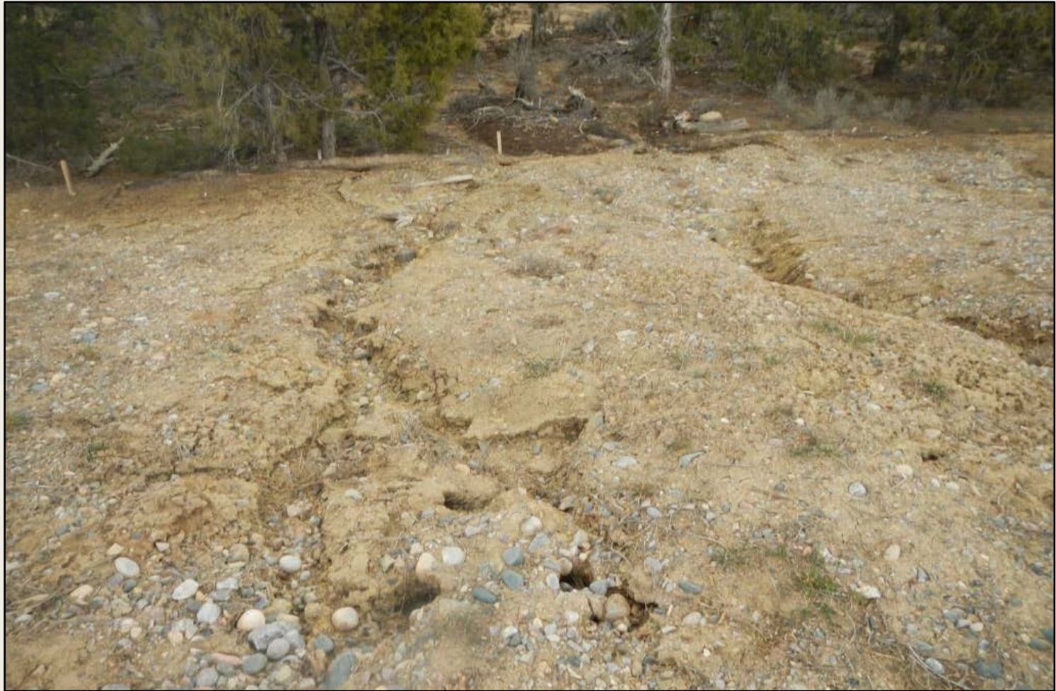
Photo 3. View of erosional channels and failed wattles within the eastern project area.
