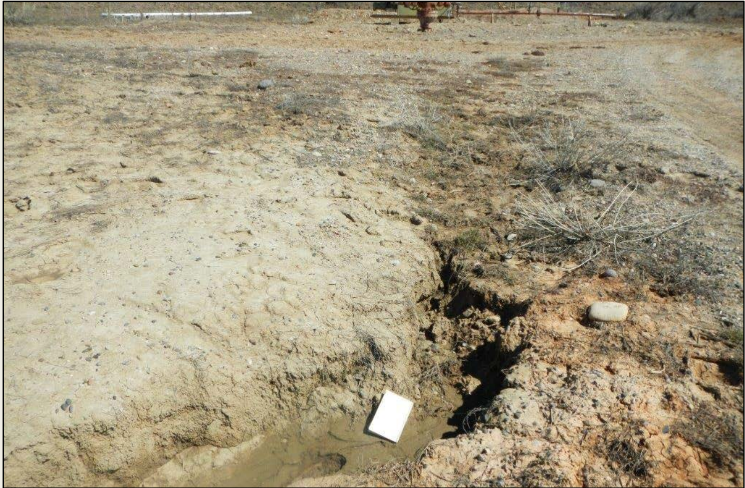
Photo 2. View of headcut erosion approximately 2.5 feet wide and deep within the southwestern project area.
