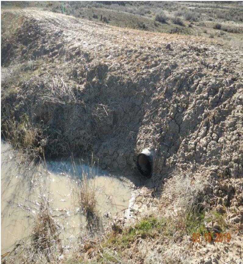
Photo#7: Overflow point of pond; South side of berm.
