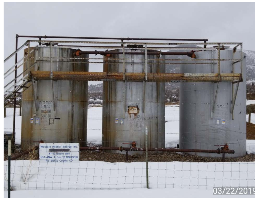
Photo 2. Tank battery.
