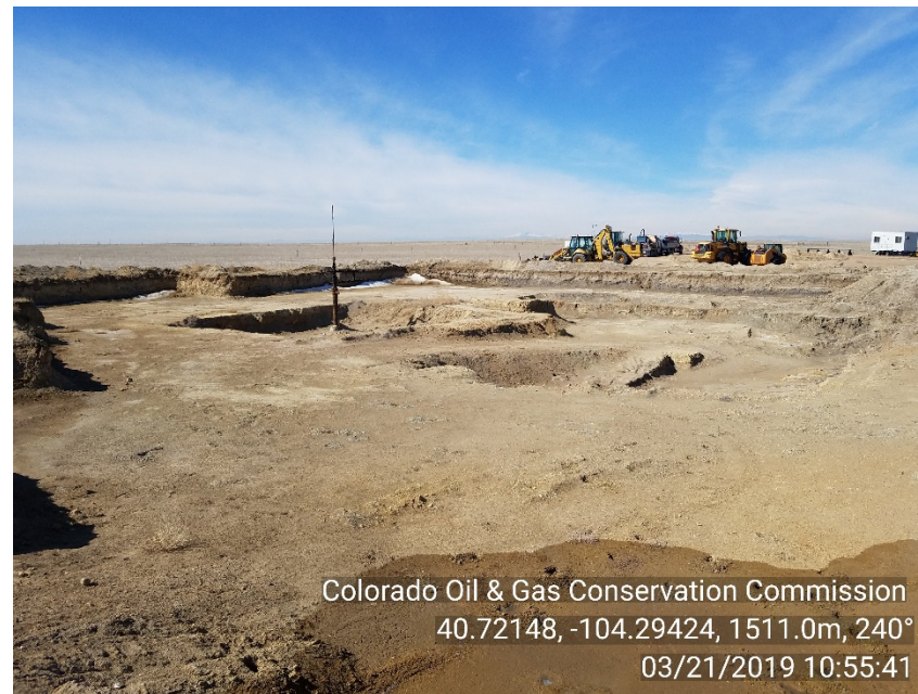
Open excavation around wellhead
