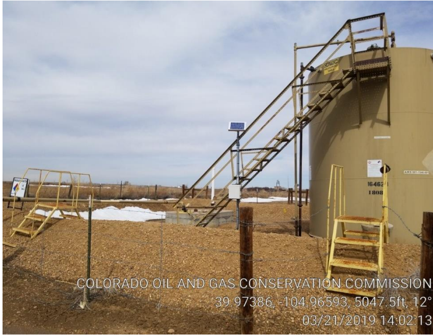
Pic 7 No anchor on tank. In flood plain.
