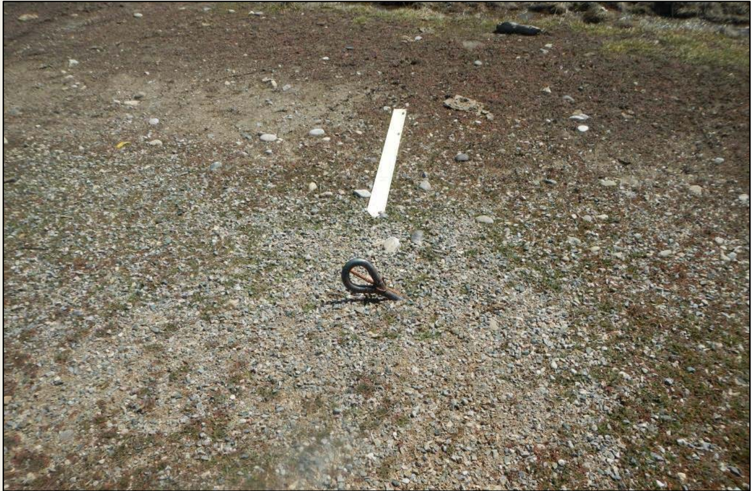
Photo 3. View of unmarked rig anchor within the project area.
