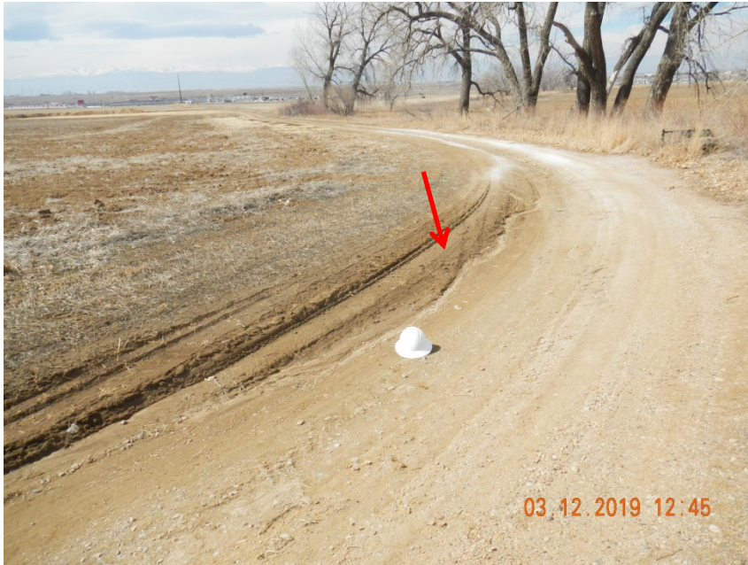
Photo 5. Photo taken from the access road, facing Northwest. Appears there is erosion along the west edge of the access road.
