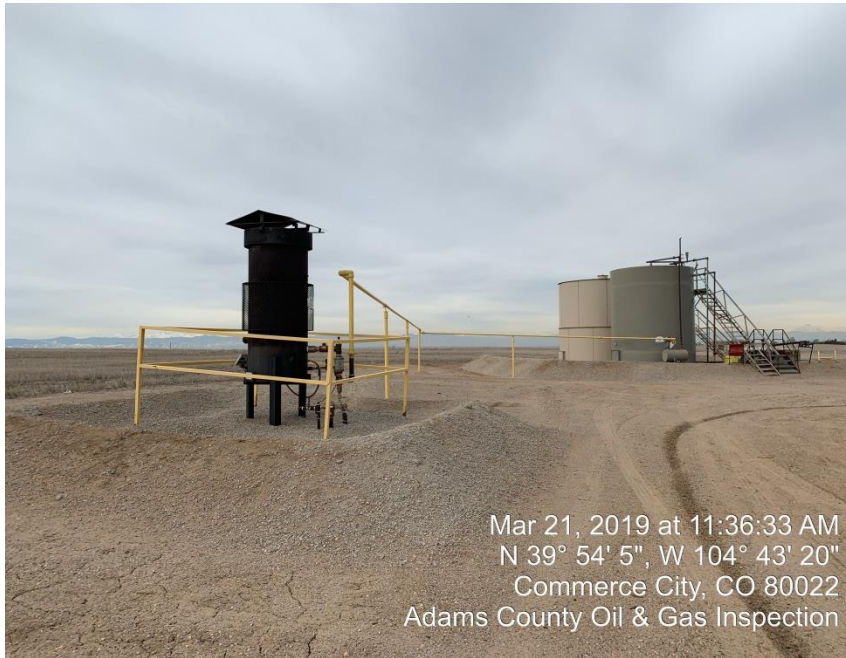
Photo#1ECD/Production Tanks/Produced Water Pit
