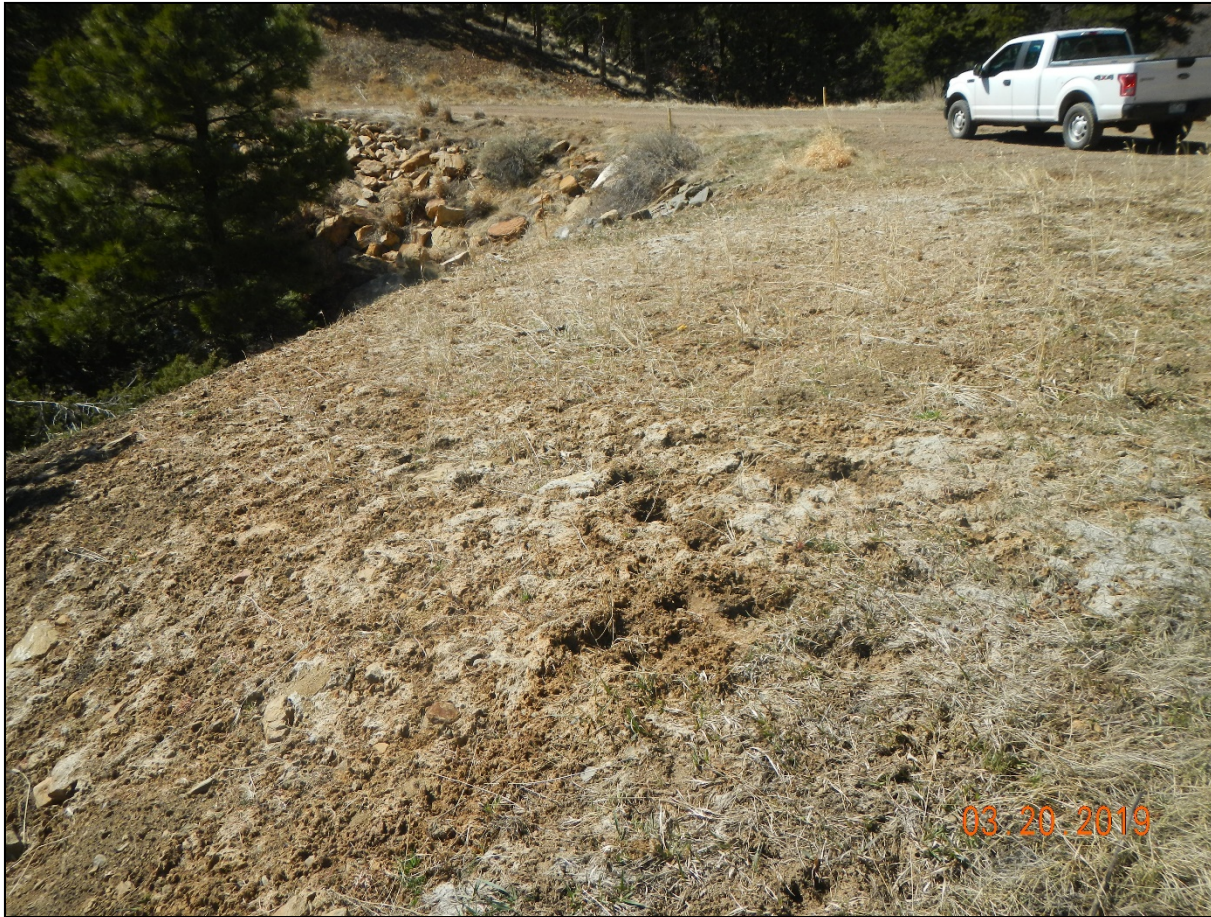
Photo 3. Gravel has been removed and disturbance reclaimed.
