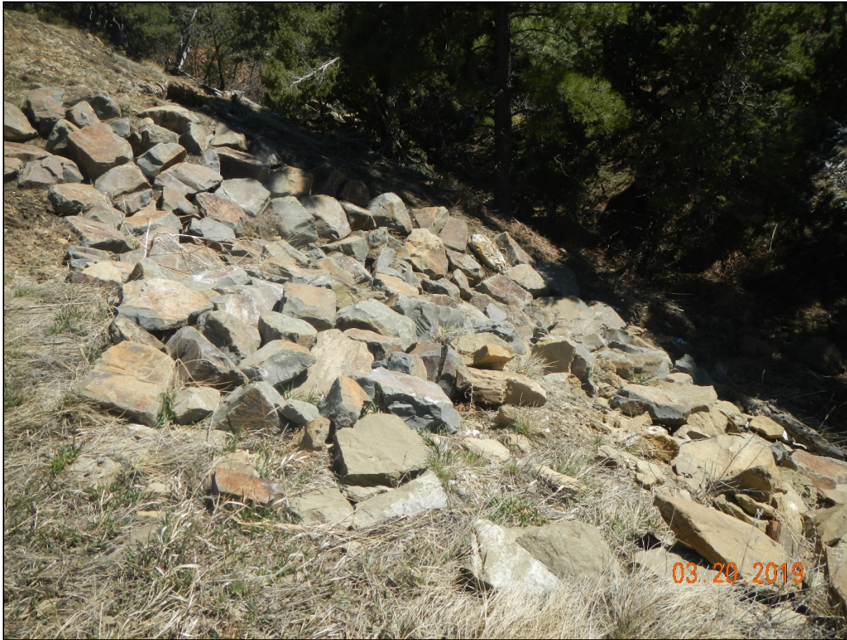
Photo 2. Rock rip/rap has been placed along the side for erosion control.
