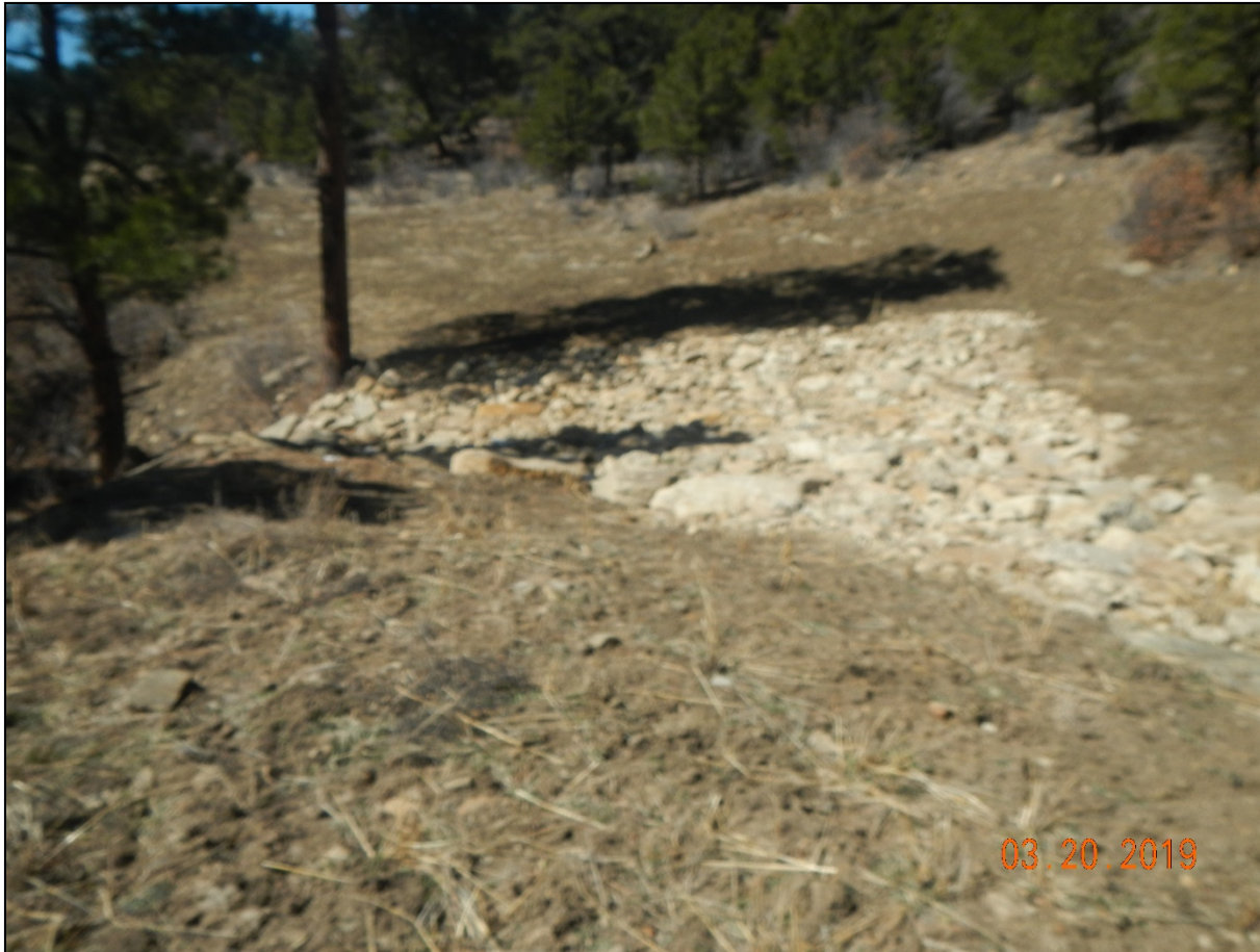
Photo 1. Facing toward the beginning of the reclaimed access road. Rock rip/rap has been placed in the drainage channel for erosion control.
