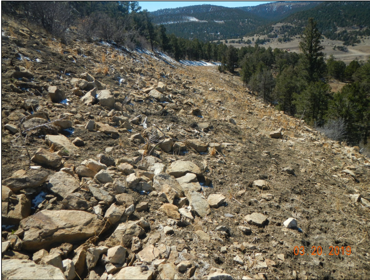
Photo 4. Facing southwest along the steep grade of the reclaimed road.
