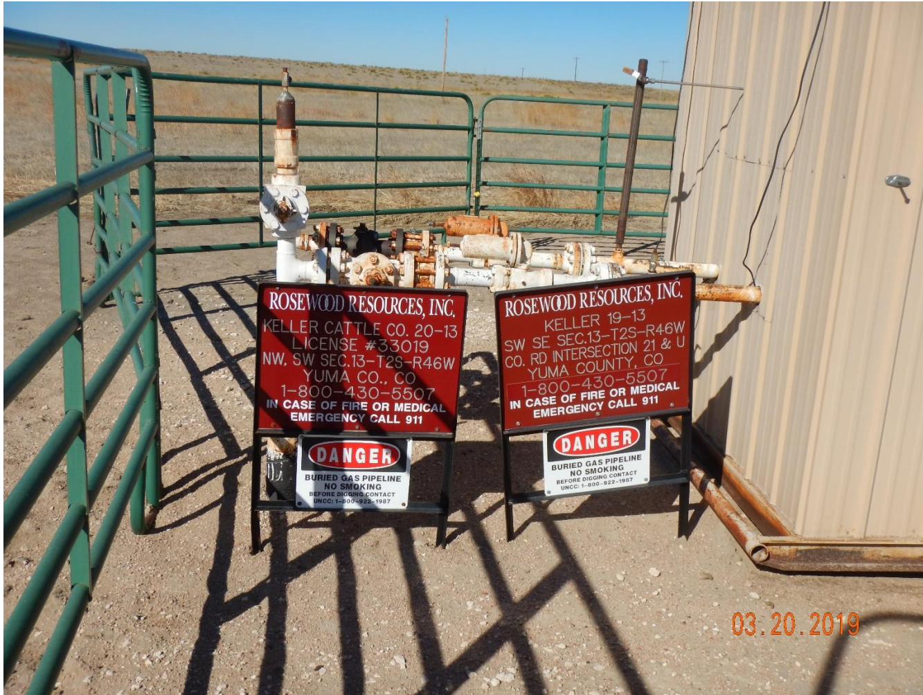
Photo 2: Photo of Rosewood signs and equipment.
