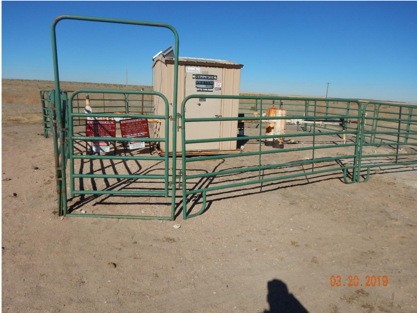
Photo 1: Photo taken from the east end of the location, facing west. Photo shows equipment remaining on location.
