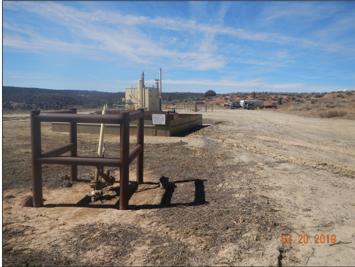
Photo of location
