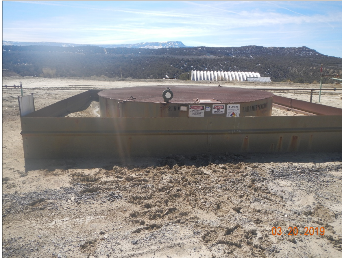
Photo of Tank Battery
