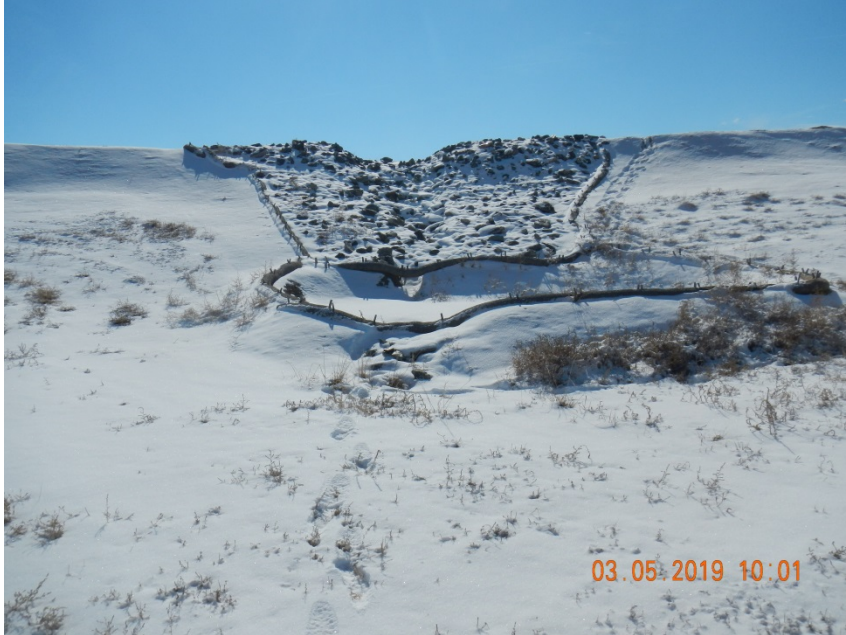
Photo 5. Photo taken from the location, facing East. See comments from Photo 4. At the time of this inspection, it appears the Operator has installed sufficient stormwater and erosion control BMPs in accordance to Rule 1002.f. standards.
