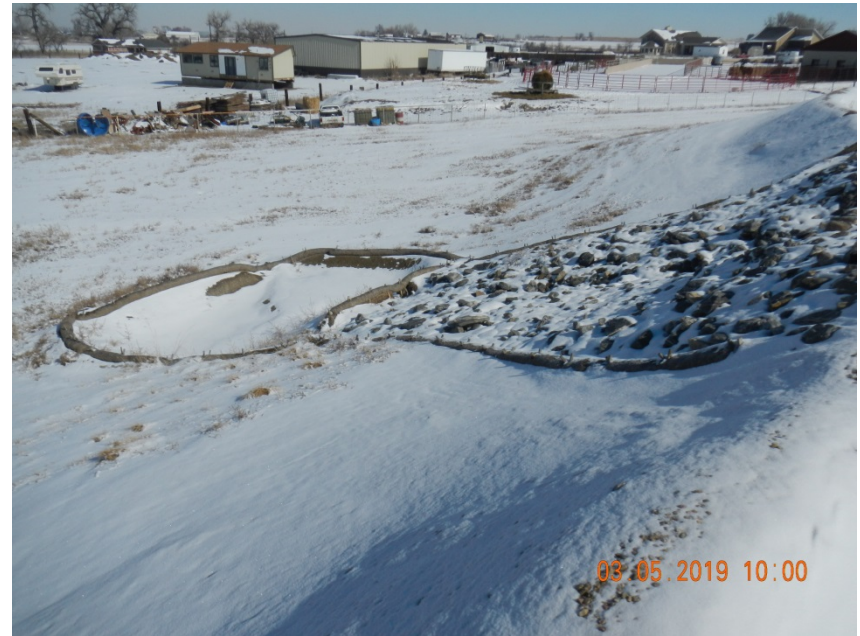
Photo 4. Photo taken from the northwestern perimeter of the location, facing North. Appears the Operator installed sediment trap with a temporary stabilized outlet.
