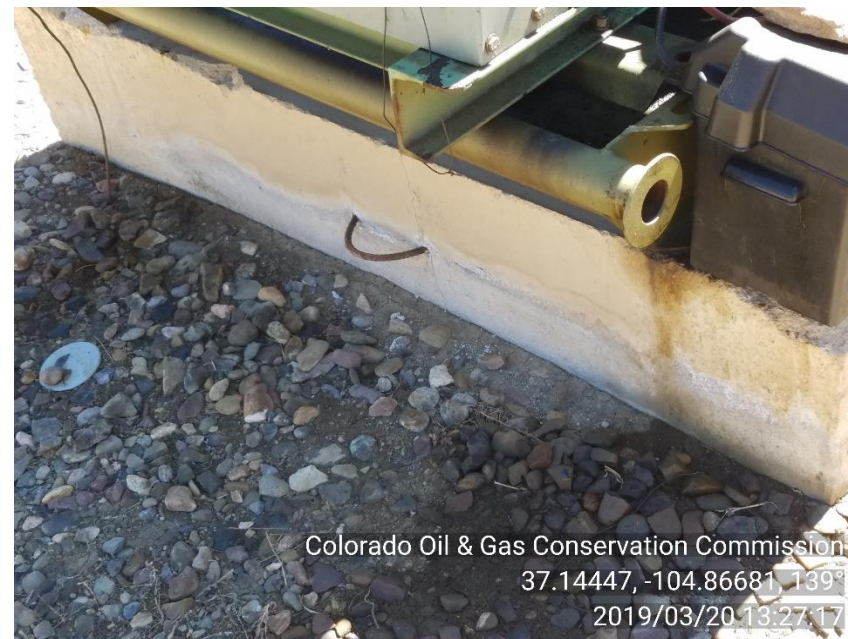
PHOTO 4: ANOTHER PHOTO OF IMPACTED SOIL AROUND ENGINE SKID.
