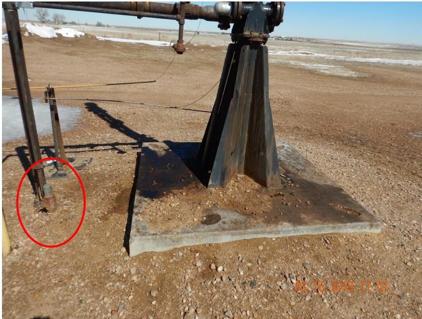
Photo 7. Photo taken from the flare, facing North. Operator has failed to inspect at regular intervals and maintain in good mechanical condition per Rule 605.d. Also, unused riser observed.
