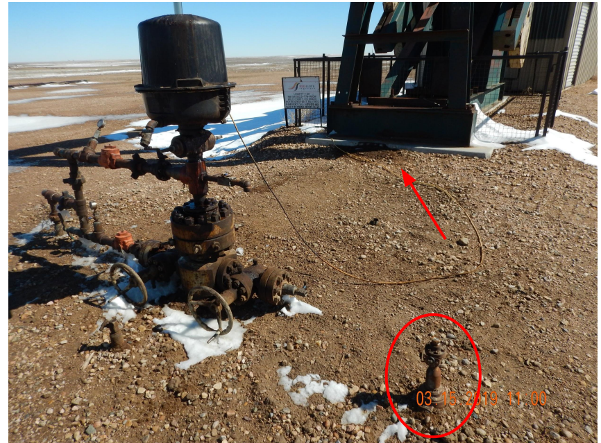
Photo 6. Photo taken from the wellhead, facing East. Appears the Operator has cleaned stained soil around the wellhead but has failed to remove the unused riser and stained soil was observed at the base of the pumpjack.
