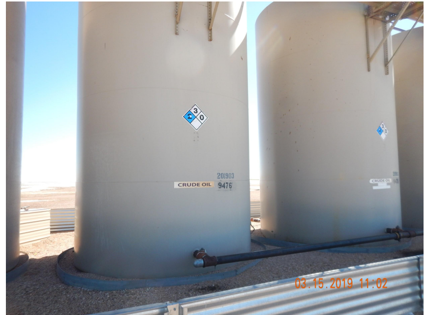
Photo 10. Photo taken from the production tanks, facing East. Operator has failed to perform the previous corrective action. No capacities on production tanks.
