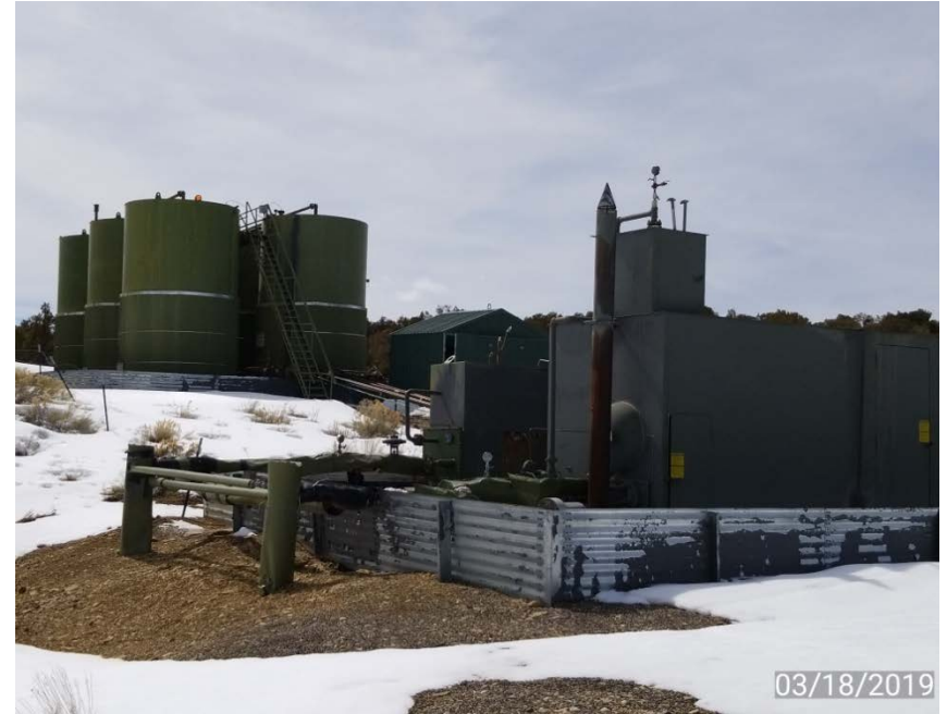
Photo 2. Separator and tank battery.
