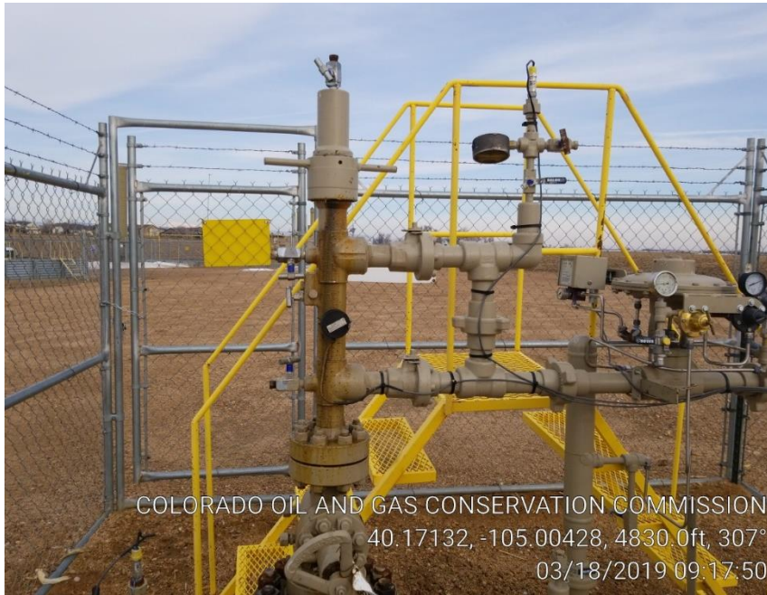
Pic 9. Possible leak on lubricator cap.
