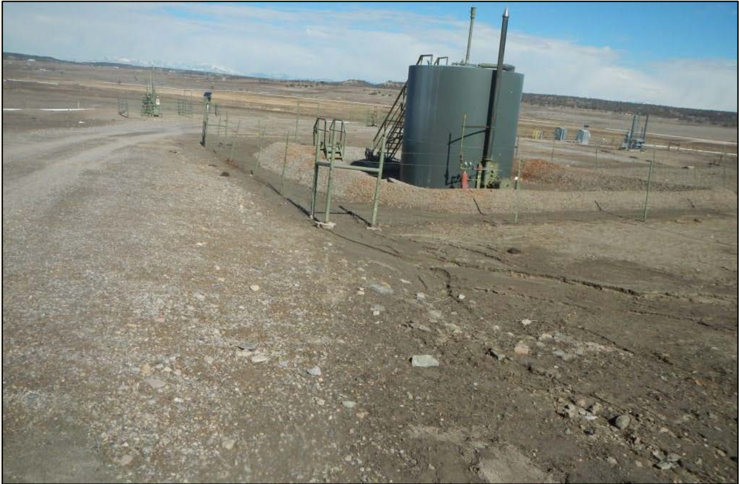
Photo 7. View of erosion occurring along the access road and onto the project area within the southeastern project area.
