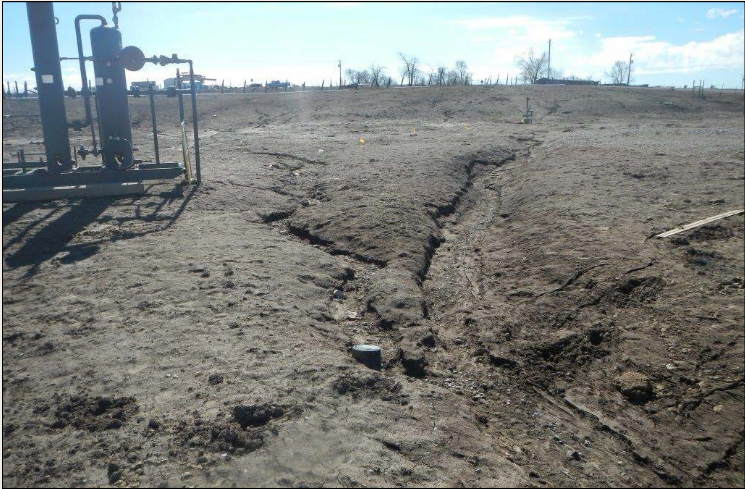
Photo 1. View of the northern project area from the northern edge of the driving surface facing eastward. An erosional channel that is approximately 2-4 feet wide and 2 feet deep is eroding the northern project area.
