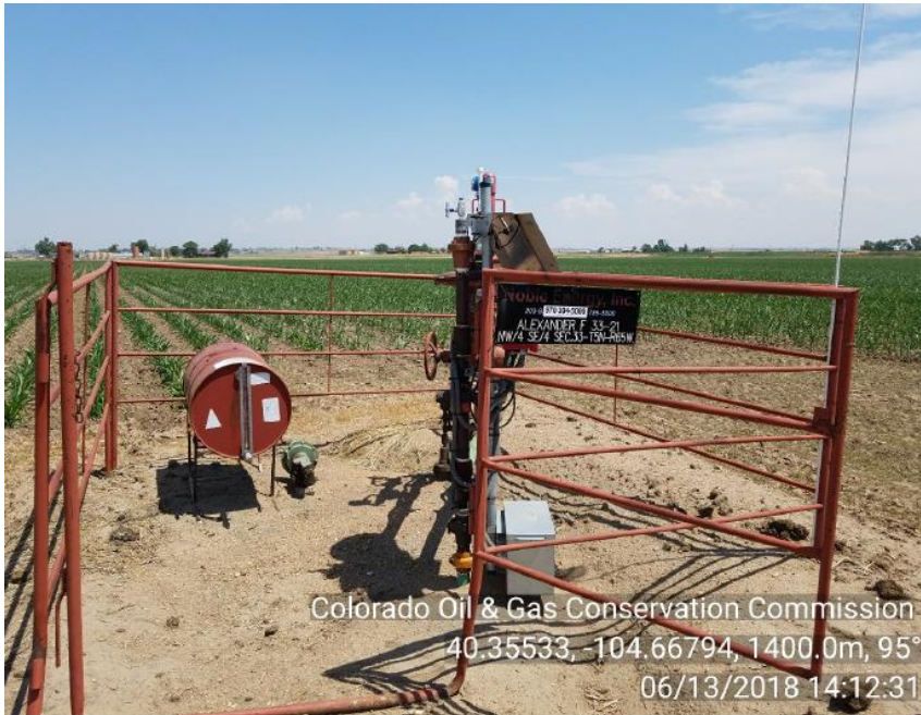
Photo 1: Previous inspection photo
