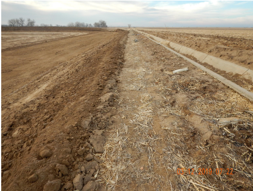
Photo 3. Photo taken from the northwestern location, facing South. Photo illustrates a berm BMP which has been installed along the western perimeter of the location. Berm BMP appears to be unconsolidated along portions of the location. An unconsolidated berm BMP is not a proper functioning BMP.
