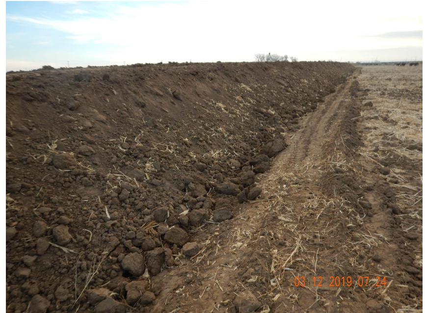
Photo 4. Photo taken from the southwestern location, facing East. Photo illustrates the topsoil stockpile. Also, the ditch BMP has topsoil which needs to be cleared out and the berm BMP needs to be re-installed, as it doesn't appear to be built to a sufficient height.
