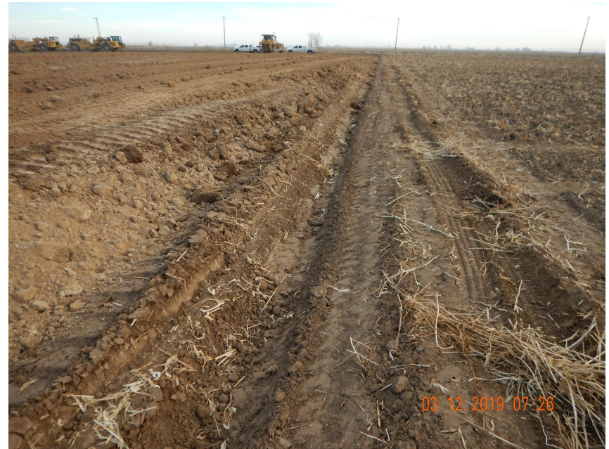
Photo 6. Photo taken from the southeastern location, facing North. Photo illustrates a ditch and berm BMP. Berm BMP needs to be re-installed, as it doesn't appear to be built to a sufficient height.
