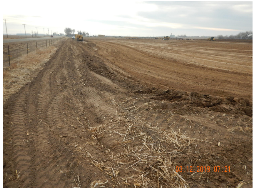
Photo 2. Photo taken from the northwestern location, facing East. Photo illustrates a ditch and berm BMP.
