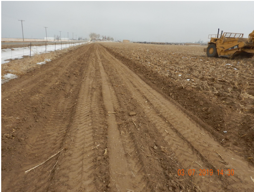
Photo 1. Photo taken from the northwest perimeter of the location, facing East. Photo illustrates a ditch and berm BMP which has been installed around the entire perimeter of the location.
