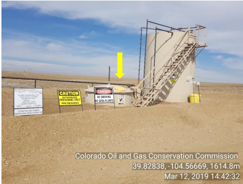
Photo 3 Hatch on H2O tank has been installed
