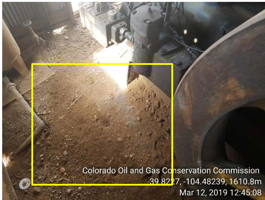
Photo 3 Stained soil inside PU motor house
