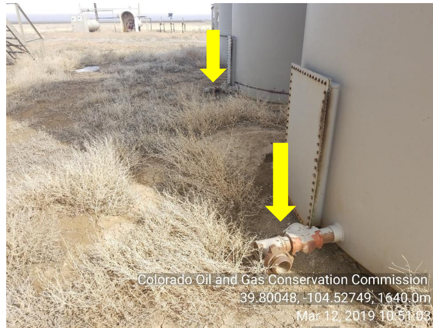
Photo 10 Crude oil tanks have no bullplugs on load lines
