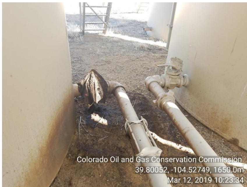
Photo 3 Mechanical and stained soil between crude oil tanks
