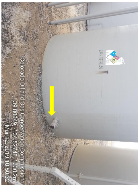
Photo 9 H 2 O production tank has no bullplug on load out line.
