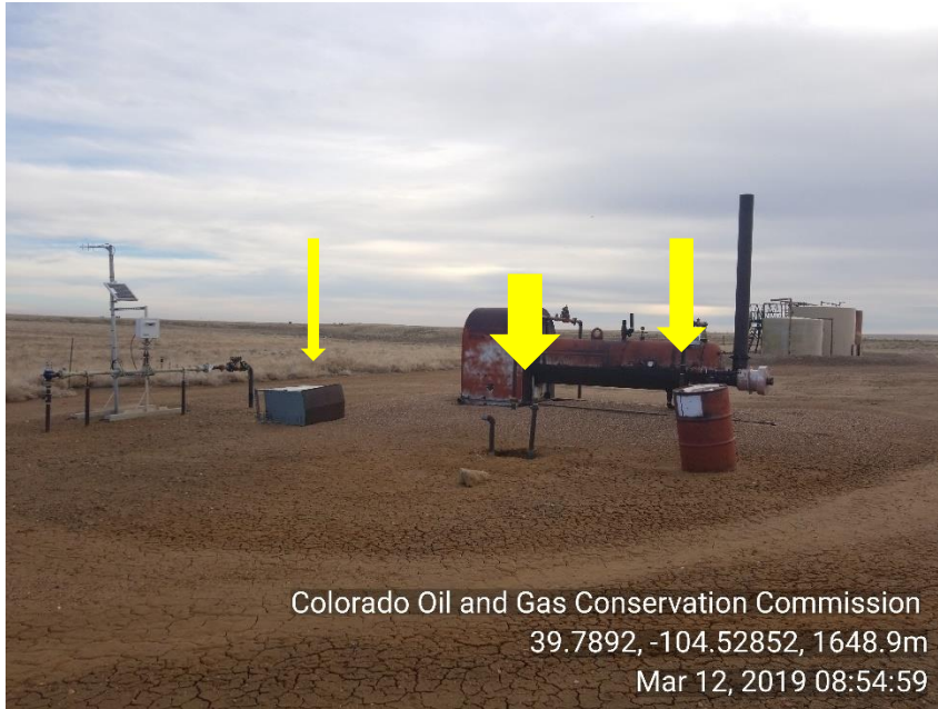
Photo 3 Meter run and separator. Unused equipment 55gal drum and meter run box. Unused unmarked 2"risers.
