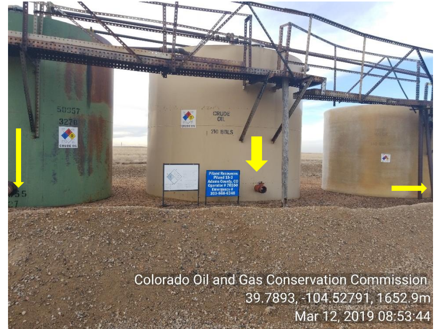
Photo 2 TNK BTRY load lines not bull plugged
