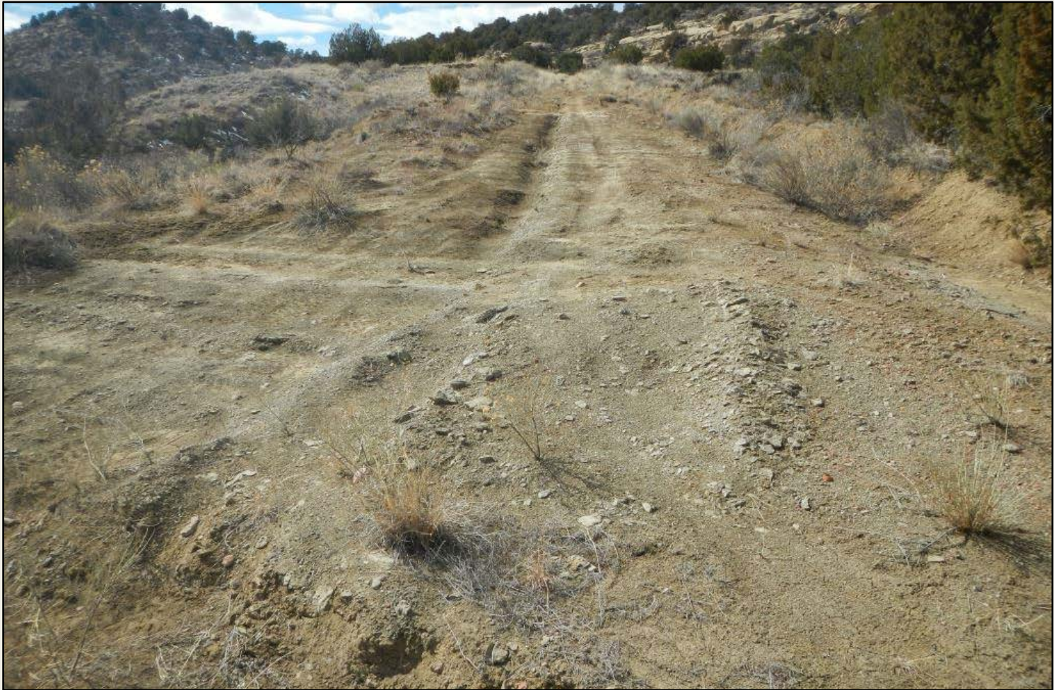
Photo 1. View of the access road from the beginning of the road facing upslope toward the well pad. Access road is not reclaimed.
