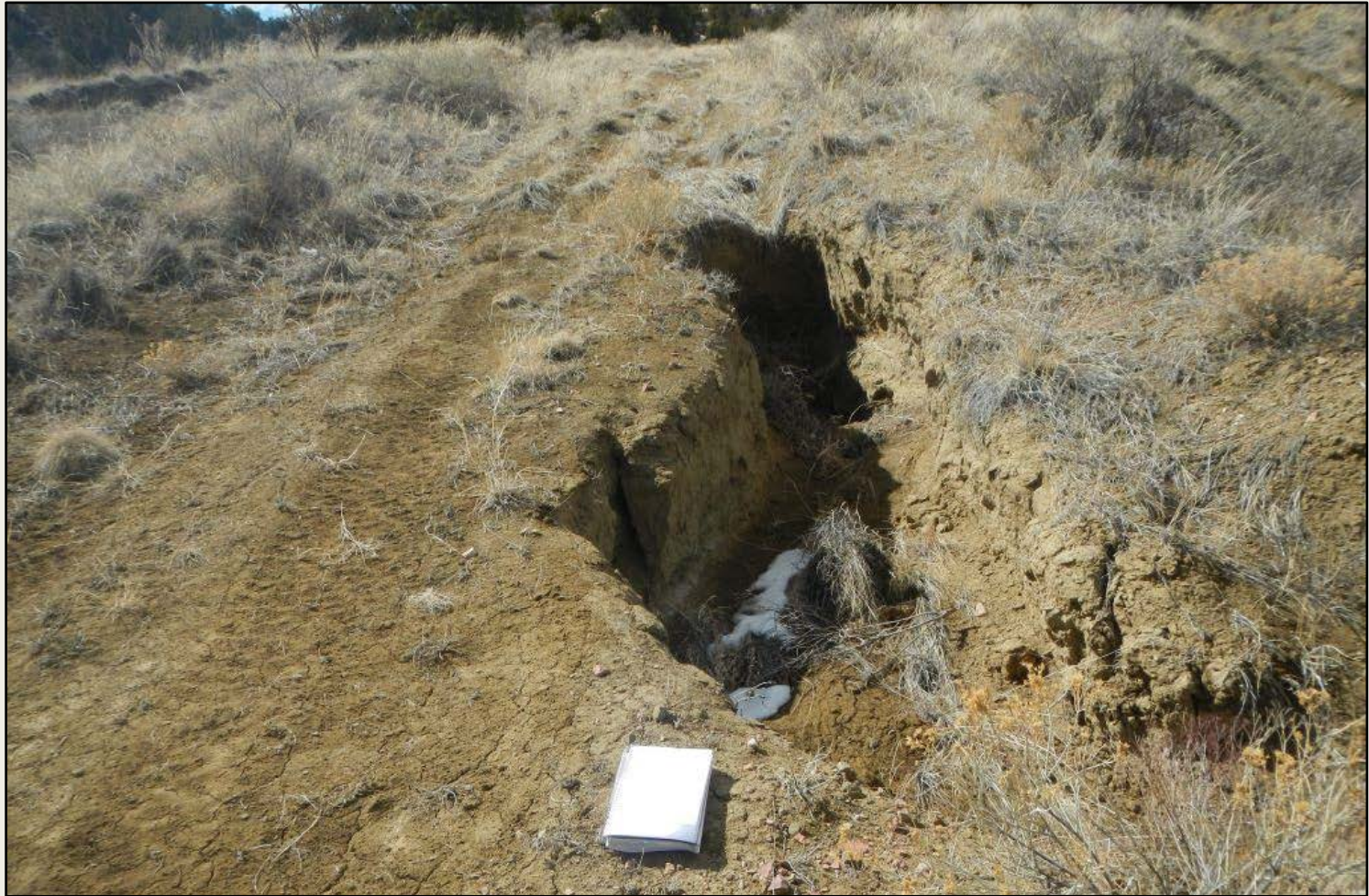
Photo 2. View of erosional headcut approximately 3-4 feet wide and deep along the access road that needs to be reclaimed.
