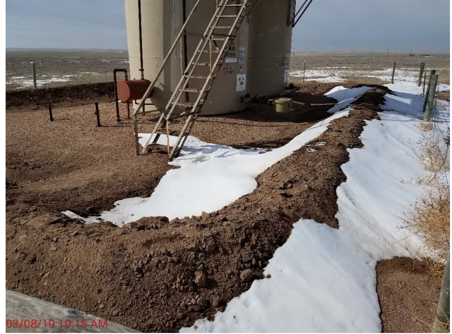
Photo 2 – Secondary containment crude oil ASTs recently graded and improved
