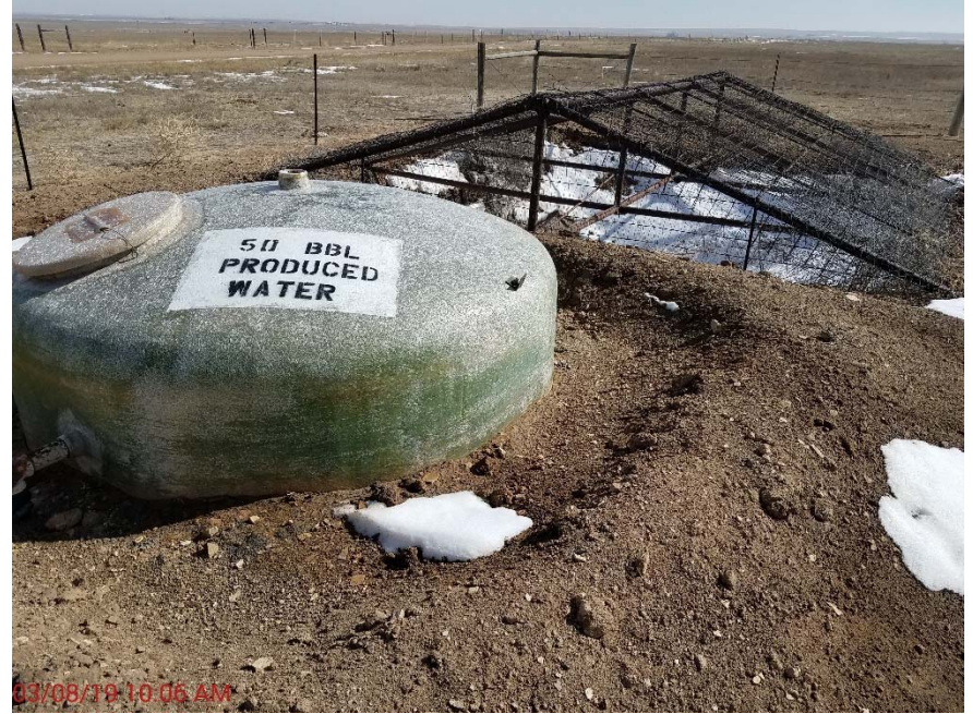
Photo 2 – Secondary containment around skim tank
