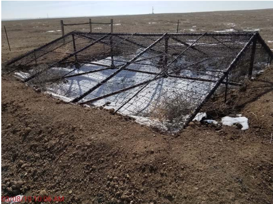
Photo 1 – Pit netting and berms improved, weeds removed.
