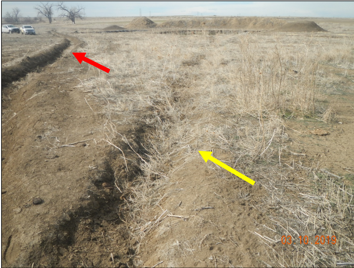
Photo 4. Facing southwest toward the location. The ditches directed toward the pit will need to be filled in and reclaimed (Yellow arrow). The ditch at the eastern perimeter (red arrow) can remain.
