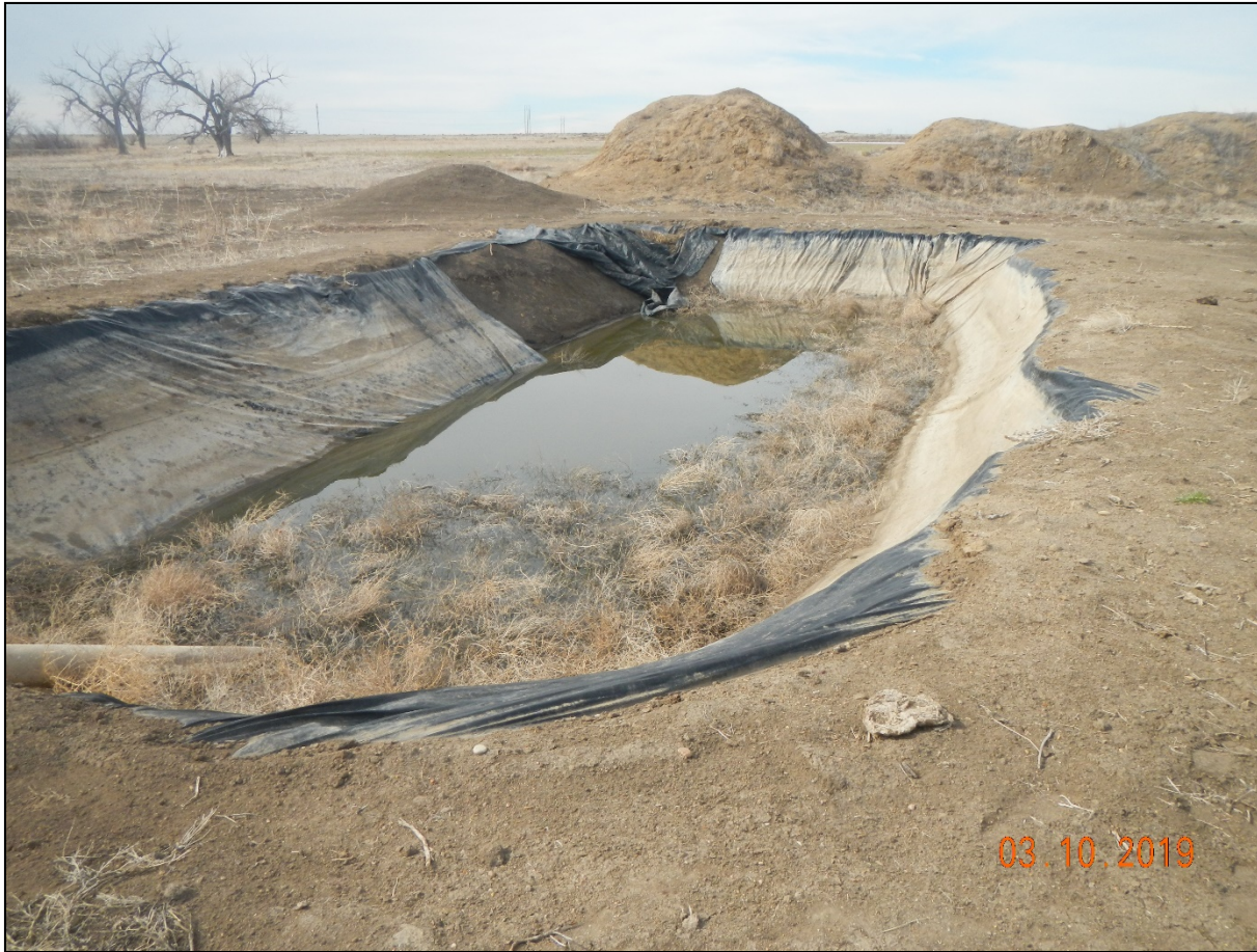
Photo 2. Pit liner remains in the south pit. The liner is torn and not maintained.
