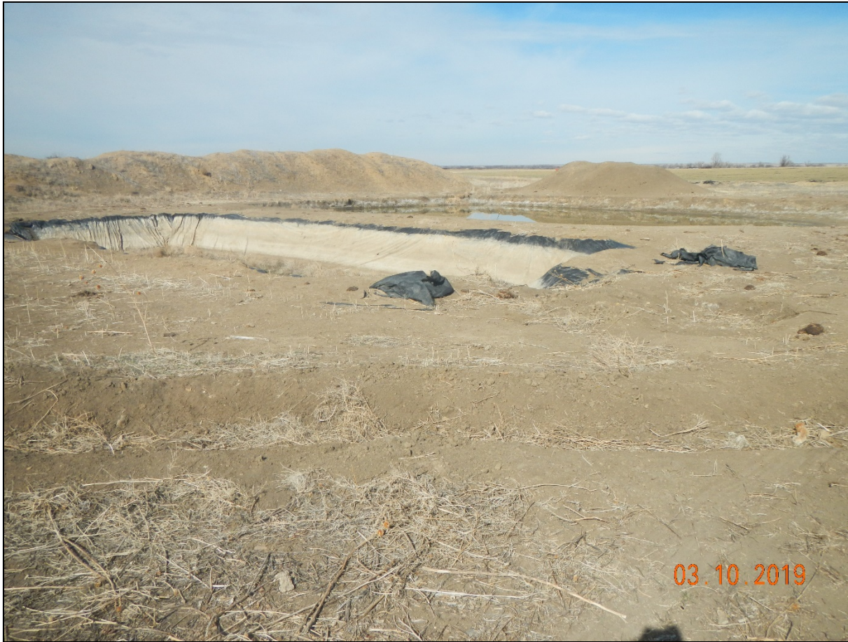
Photo 1. Facing northwest at the location. Two drilling pits remain. The location has not been recontoured and reclaimed.
