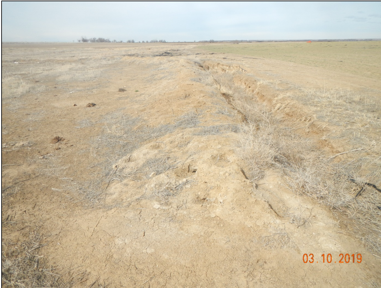
Photo 6. The northern ditch needs to be filled in and reclaimed.
