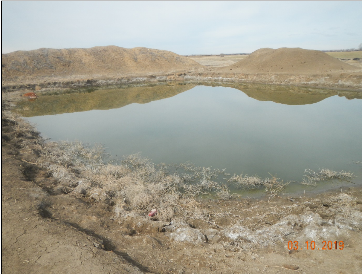
Photo 3. The north pit is full of water. Water will need to be pump out and drained.
