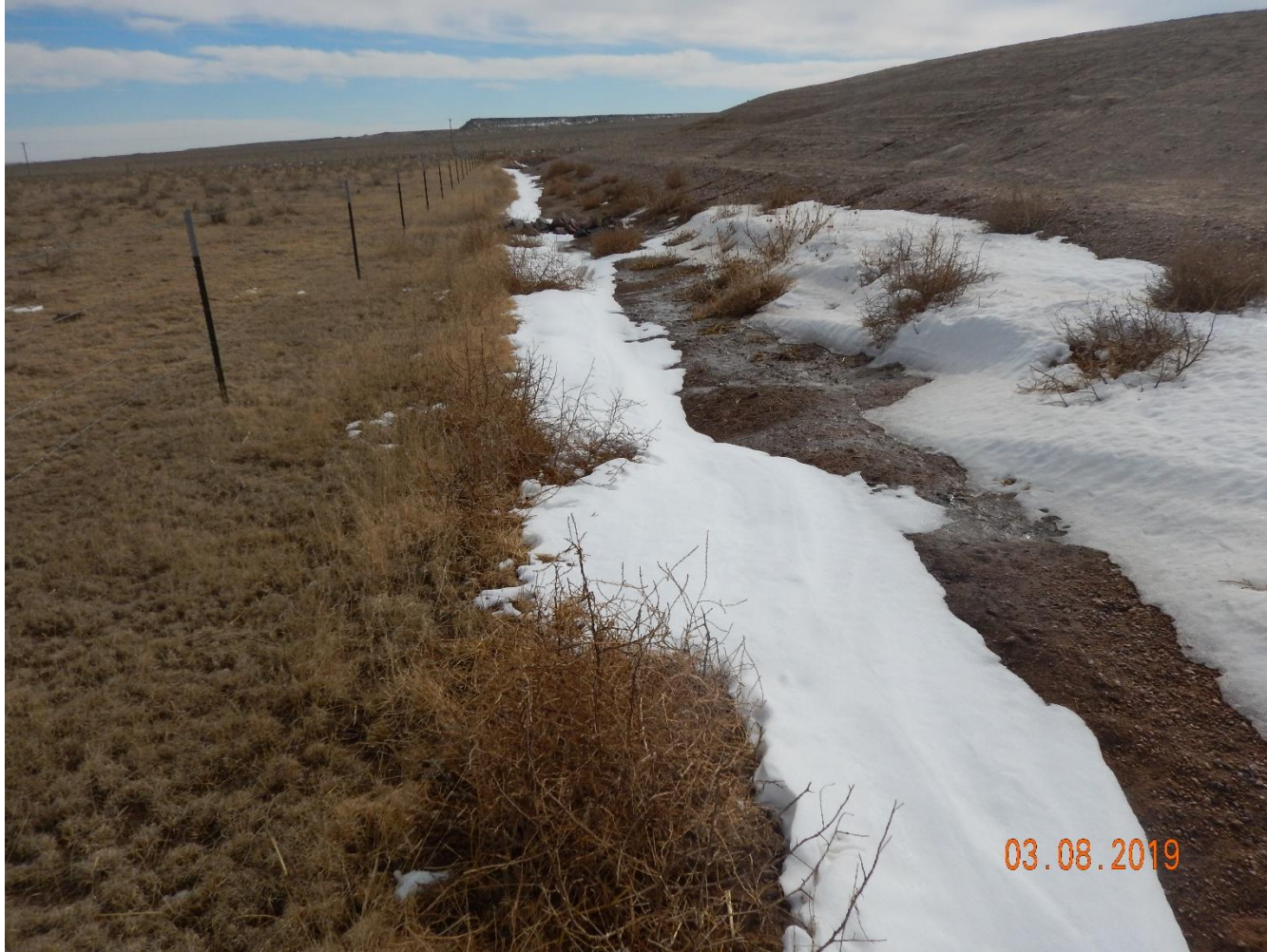
Photo 1: Photo taken from the ditch along the eastern perimeter of the location. Areas of the stormwater ditch appears to have filled with sediment. Advise maintenance.
