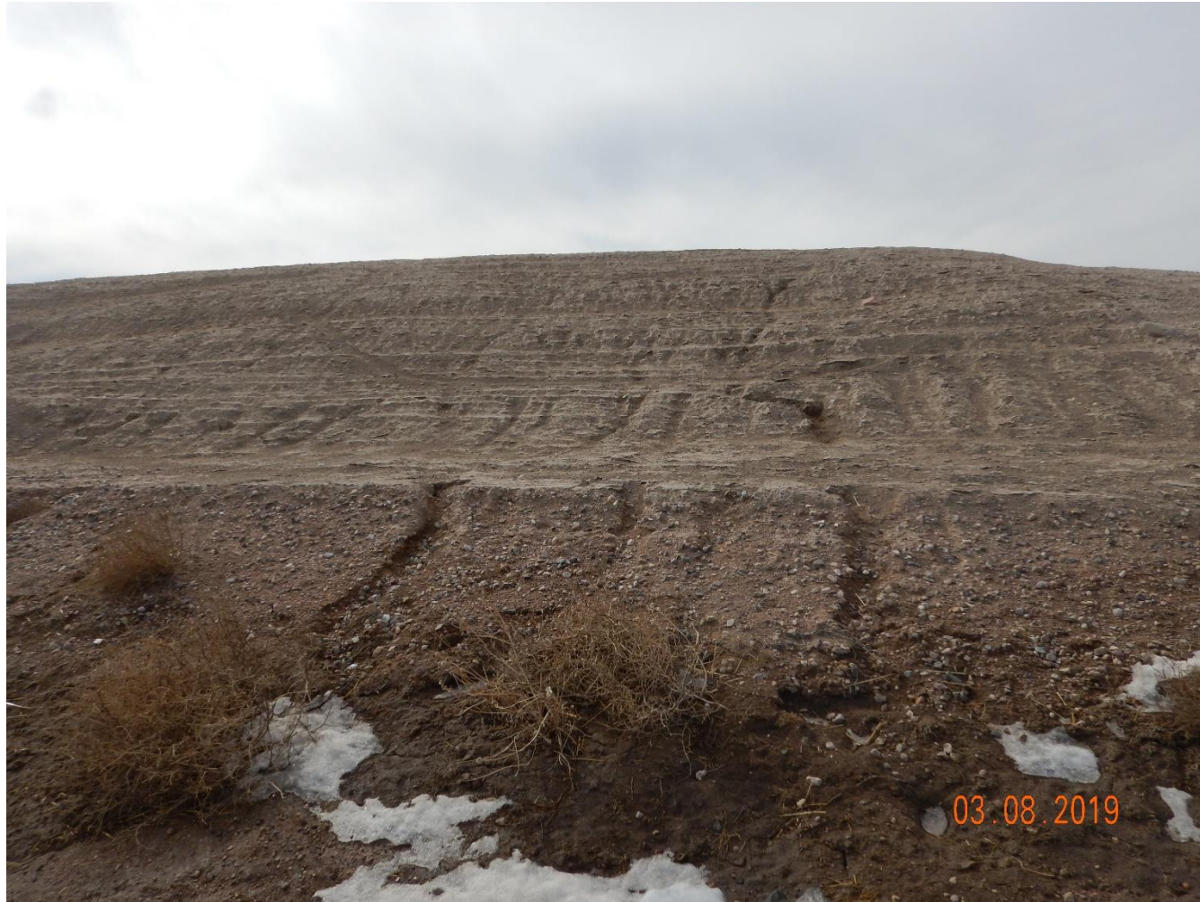
Photo 3: Photo taken from the northeast corner of the location, facing west. Photo shows erosion degradation on the soil stockpile.
