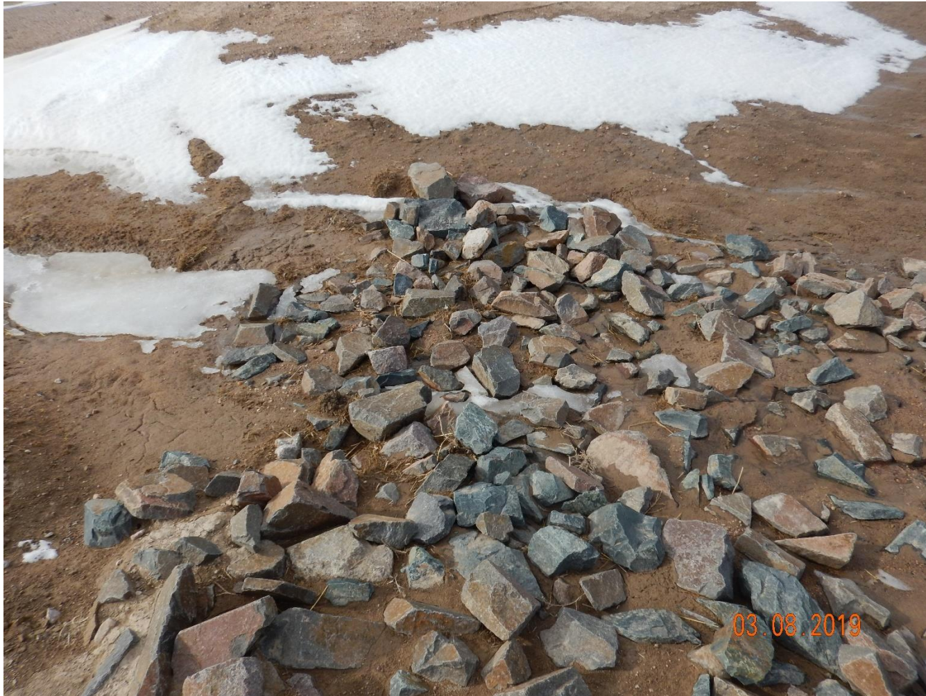
Photo 8: Photo taken from southwest corner of the sediment trap. Photo shows inlet is filling with sediment. Advise maintenance.
