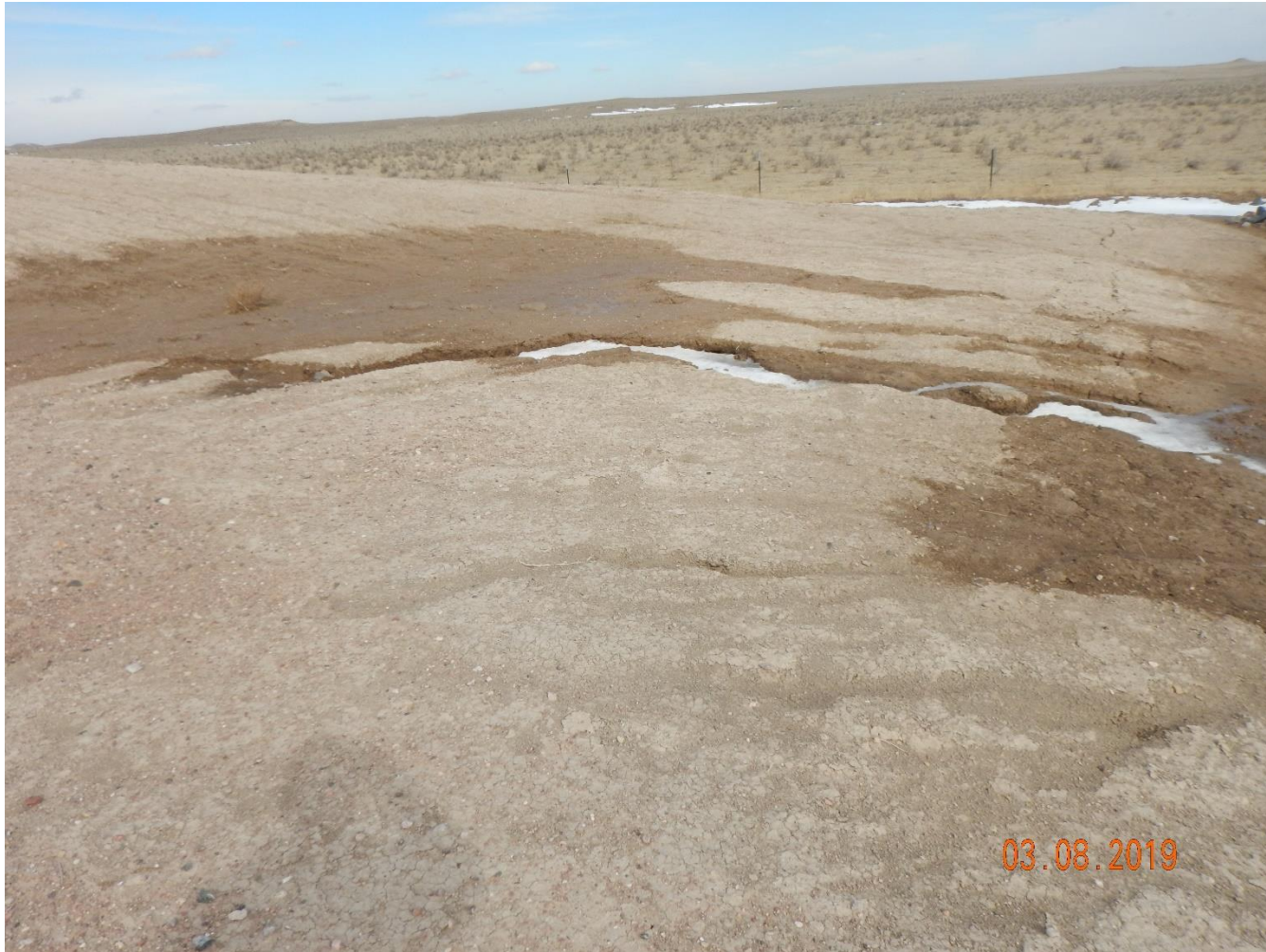
Photo 6: Photo taken from northwest corner of the sediment trap. Photo shows insufficient inlet protection. Gully erosion evident at trap.
