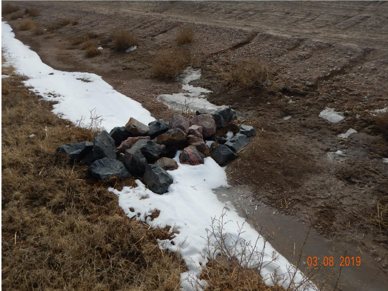
Photo 2: Velocity checks within stormwater ditch. Erosion degradation at soil stockpile.
