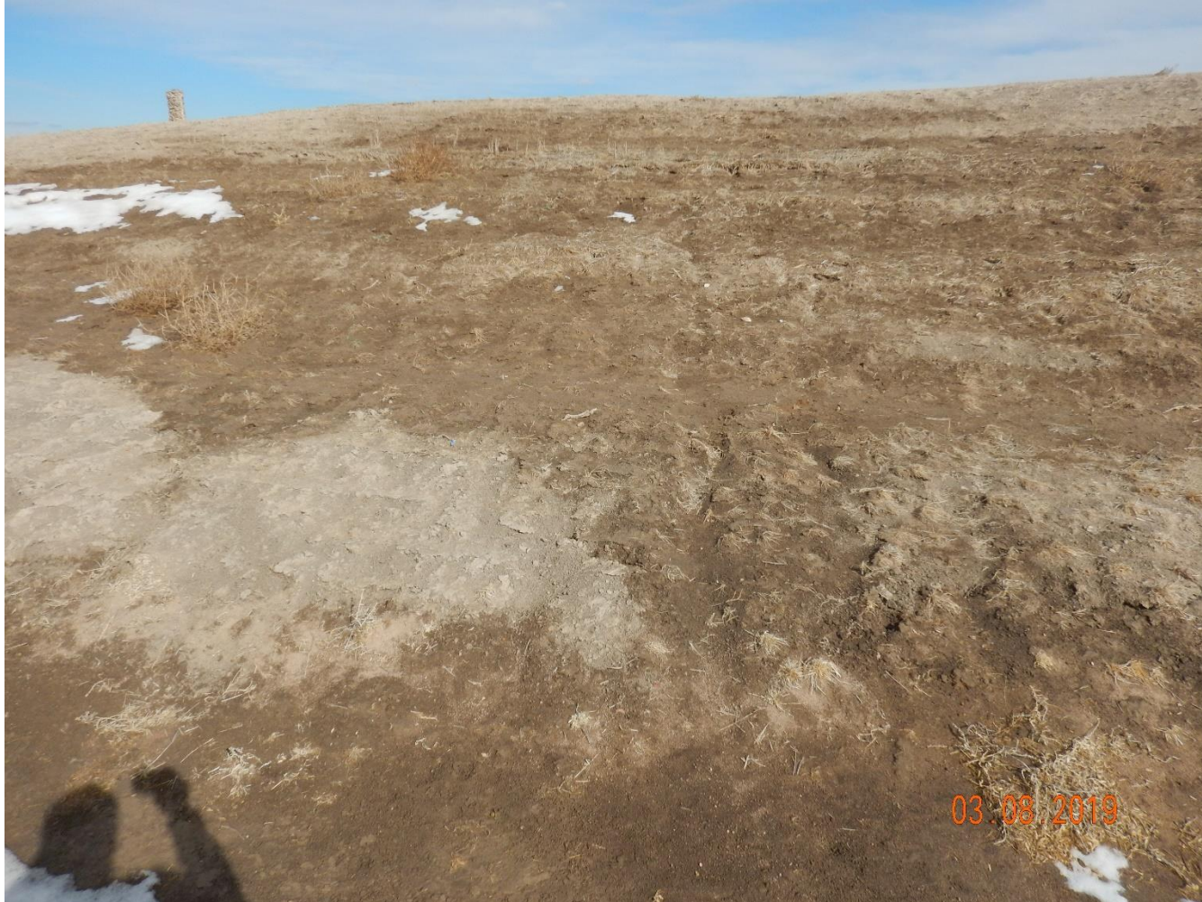
Photo 10: Photo taken from topsoil stockpile on the east end of the location. Photo shows stormwater degradation becoming evident.
