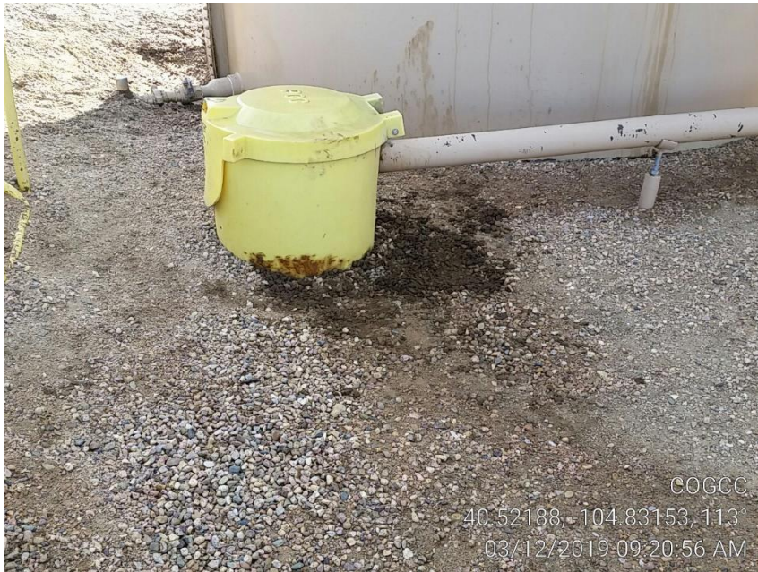
Photo 3 – Stained soil at load line bucket
