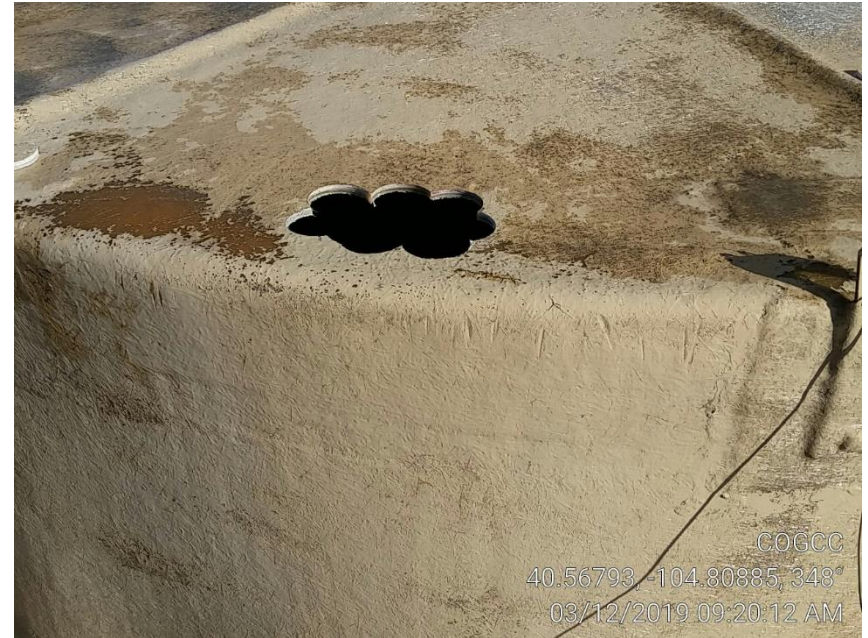
Photo 2 – Water Tank hole on top missing screen
