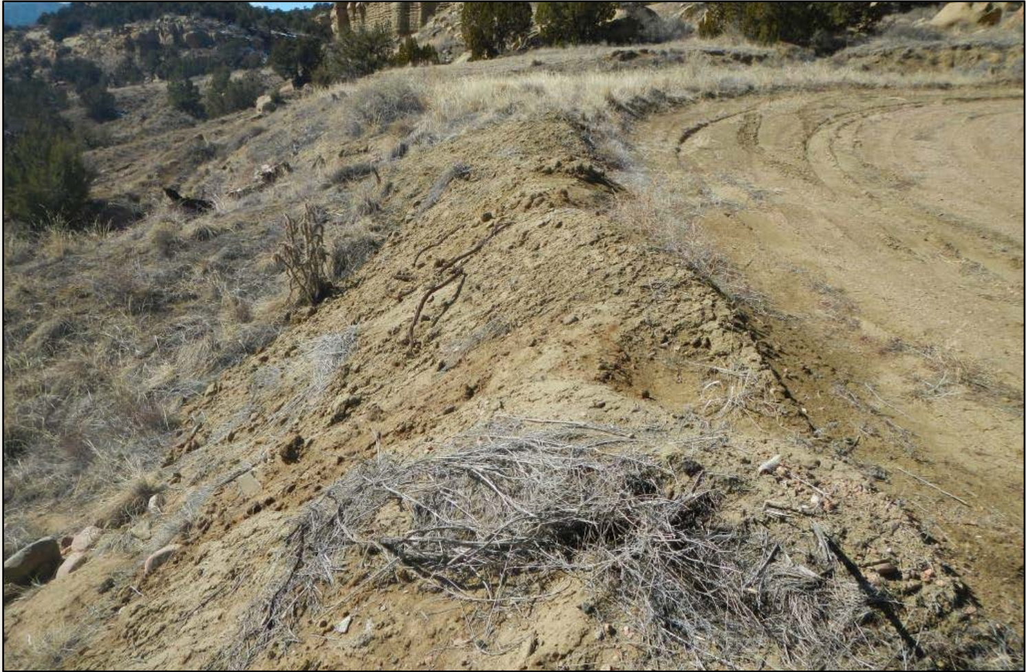
Photo 2. View of the eastern project area from the northeastern edge facing southward. Vegetation on the slope is sparse and needs stabilization. Metal cable debris is present. Loose soil on edge is insufficient to function as berm.
