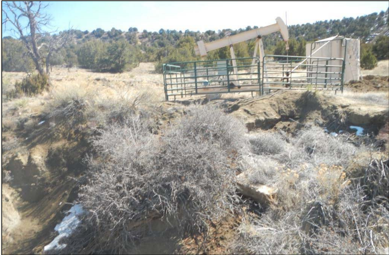
Photo 1. View of the northern project area from the northwestern edge facing toward the wellhead. Wellhead is adjacent to an erosion channel. This area needs immediate stabilization to prevent any further erosion.
