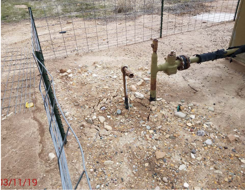
Location Photo #3, unmarked flow line riser near meter run.
